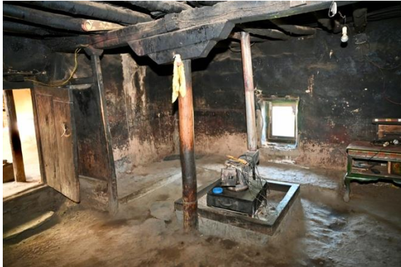
Figure 31: The caretaker's kitchen before restoration.
