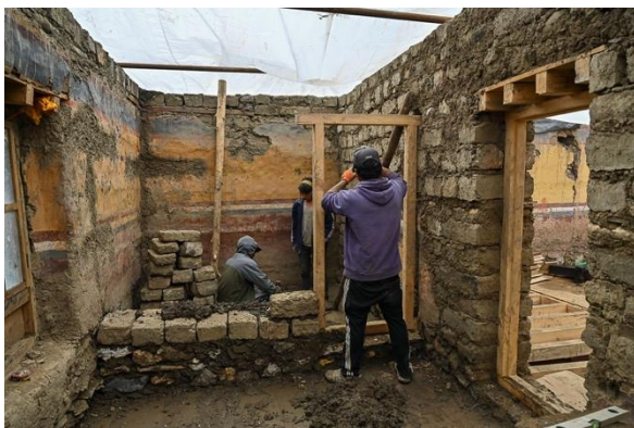
Figure 25: Construction of the new bathroom.
