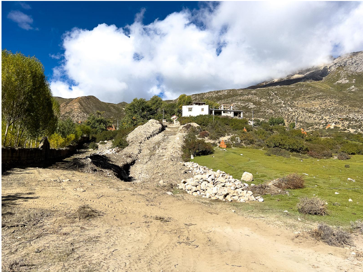
Figure 40: View from the walking path leading up to the monastery; the trench in the foreground prepares the concrete stairway, while the new concrete construction is seen in the background behind the white building.
