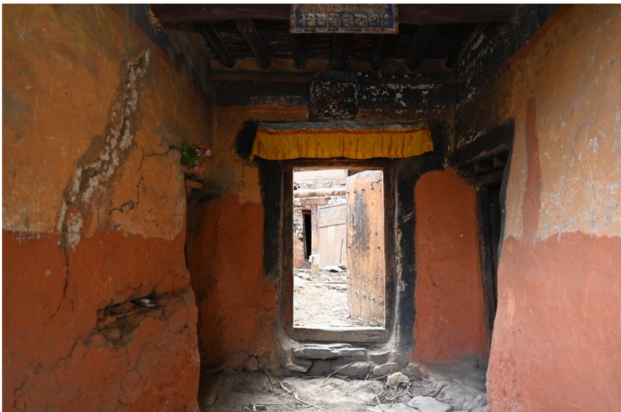
Figure 6: View of the main entry before restoration.
