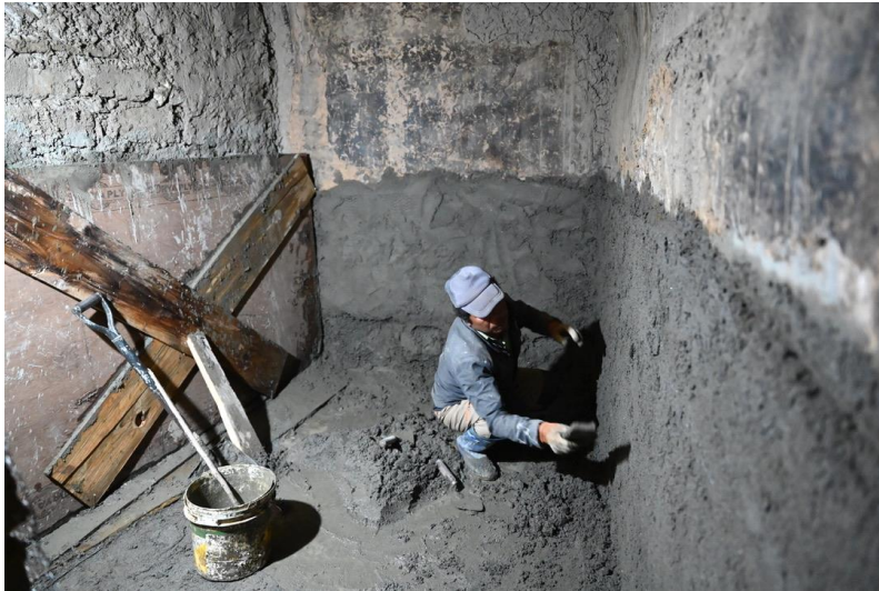
Figure 10: Rough concrete plaster applied to the lower parts of the walls of the new visitor's toilet.
