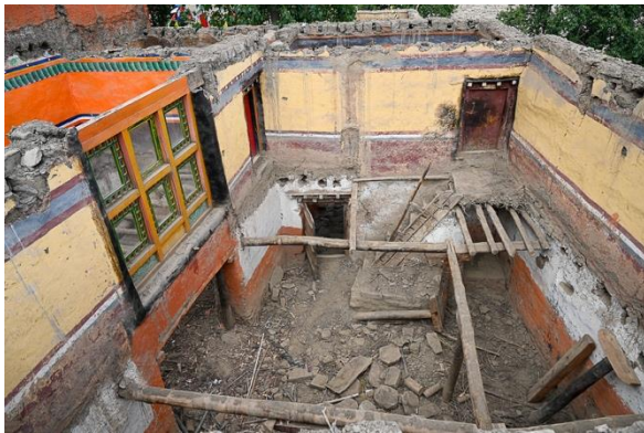
Figure 12: The atrium in the process of dismanteling.
