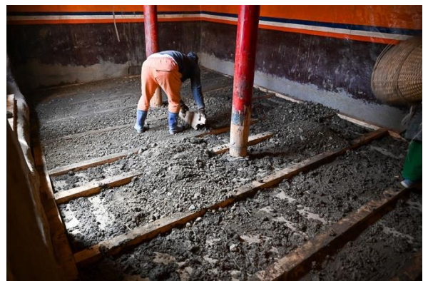
Figure 29: The installation of wooden frames in the VIP room to support the floorboards.
