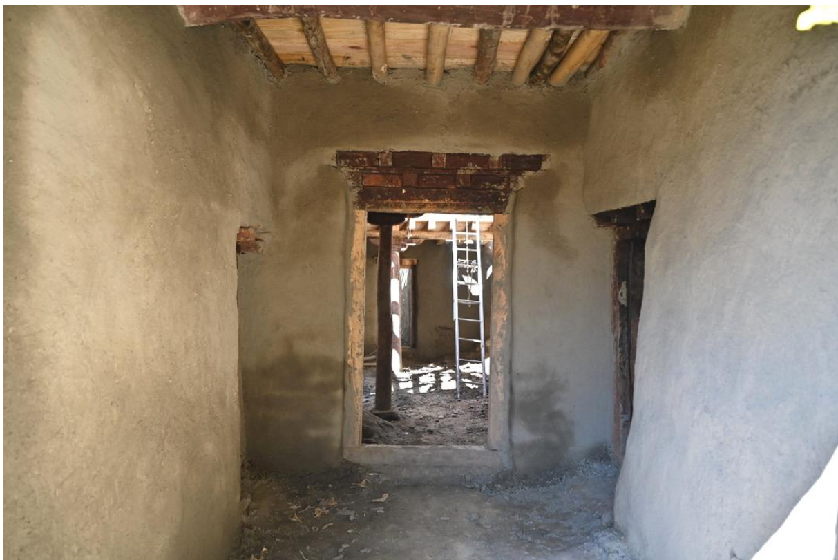
Figure 9: The main entry after the restoration of the walls with the top of the original door reused.
