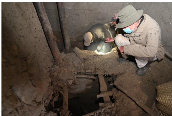
Figure 23: Surveying the space underneath the storage room.
