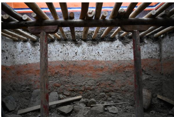
Figure 17: View into the storage room with new joists introduced.
