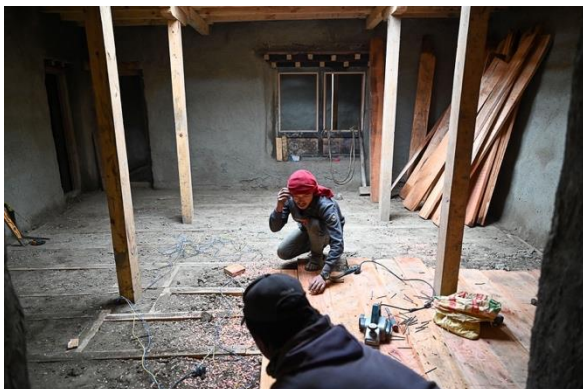
Figure 36: Installation of the wooden floor in the visitor room.
