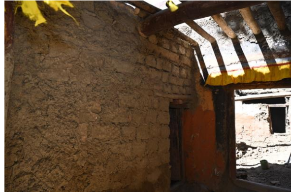
Figure 7: Left side wall before restoration, showing the stress cracks and poor foundation for the mud bricks.
