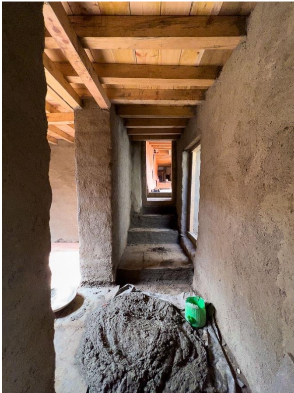
Figure 39: View of the passage to the temple with the higher walls to the guest room on the left and the door that will provide access to the roof to the right.
