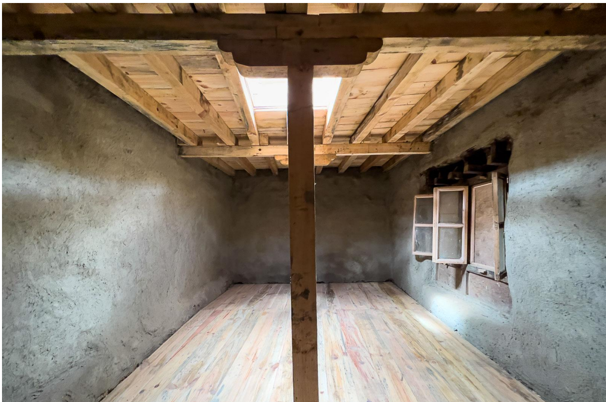
Figure 38: The restored retreat room with skylight and its original window linking this room with the guest room in front of it.
