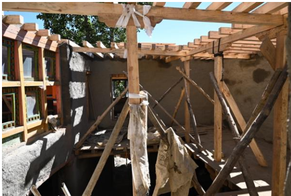
Figure 27: Construction of the upper part of the atrium.
