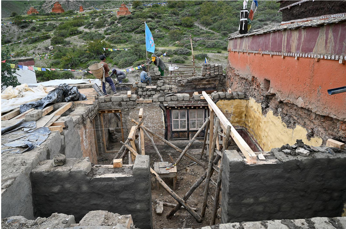
Figure 35: Restoration of the guest room with the higher walls flanking the entrance and the installation of the new beams.
