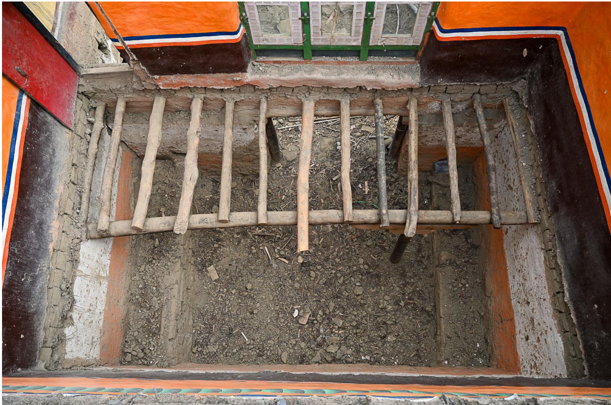
Figure 16: The former storage room underneath the VIP room seen from above during restoration.
