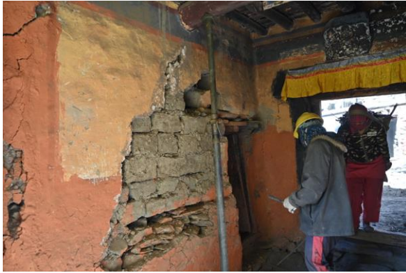
Figure 7: Left side wall before restoration, showing the stress cracks and poor foundation for the mud bricks.
