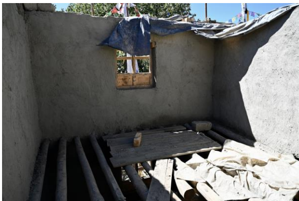
Figure 33: The caretaker's kitchen during restoration with the new window installed.
