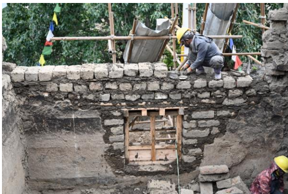
Figure 21: Introduction of the window for the visitor's kitchen.
