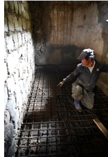
Figure 10: Rough concrete plaster applied to the lower parts of the walls of the new visitor's toilet.
