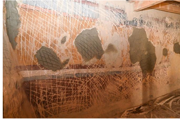
Figure 2: The Upper sanctum with the walls patched and scratched to hold the new plaster.
