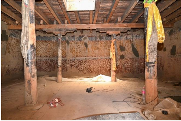
Figure 2: The Upper sanctum with the walls patched and scratched to hold the new plaster.
