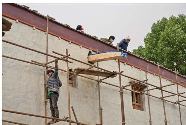
Figure 123: Installation of a new spout on the south side.
