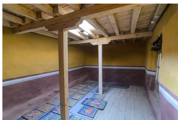
Figure 102: The same room after restoration used as a temporary storage for the stone panels of the upper sanctum.
