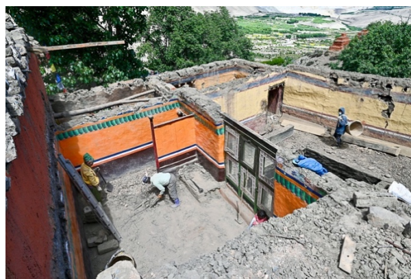
Figure 72: Removing the roof above the VIP room with the original joists exposed.
