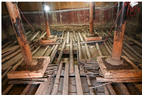
Figure 22: The wooden frames to support the bases of the pillars.
