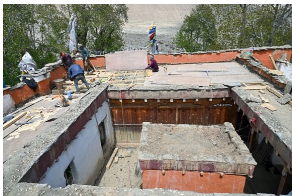
Figure 64: Constructing sloping wooden frames and installing the waterproof plywood sheets on them in May 2022.
