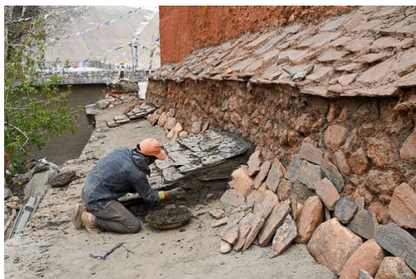
Figure 112: The roof of the mani wheel wall towards the end of the initial restoration in May 2022.
