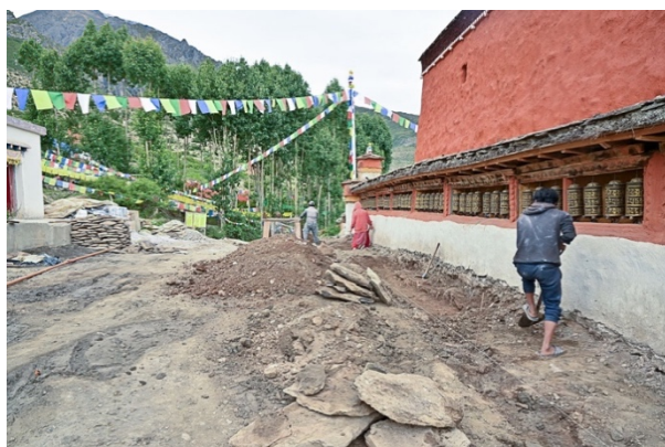
Figure 118: Work on the circumambulation path on the west side.
