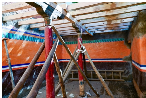
Figure 91: The new timber structure for the ceiling of the VIP room.
