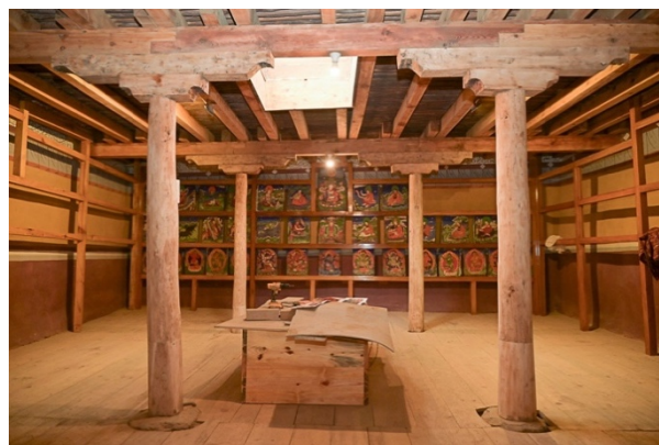
Figure 28: The Upper Sanctum after the construction of the new frames for the stone panels.
