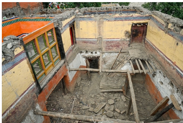
Figure 76: Deconstructing the atrium to ground floor level.
