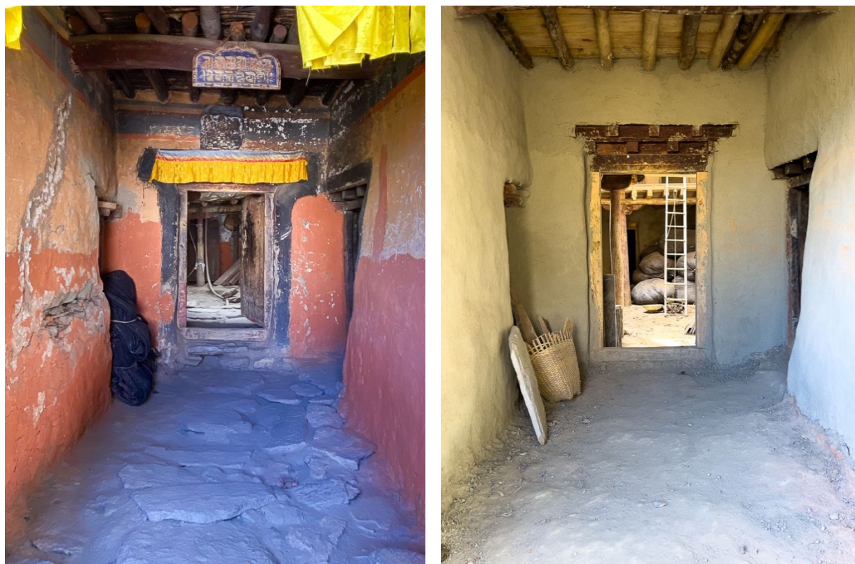
Figure 74: The entrance to the caretaker's quarter before restoration.
