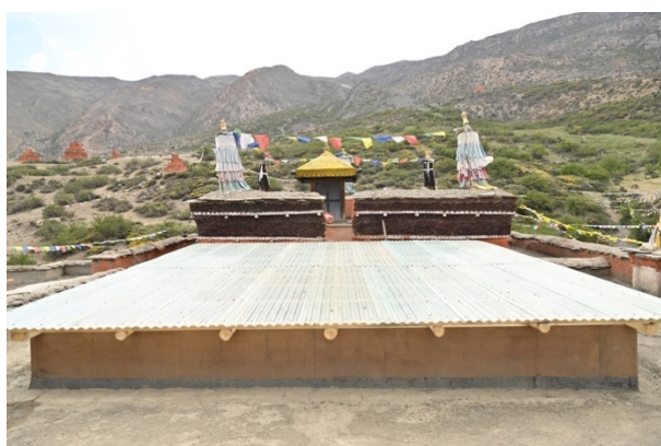
Figure 70: The roofing of the courtyard largely completed.
