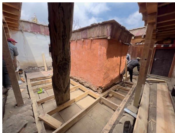
Figure 35: Adding a second wooden frame to bring the new floor to the original level.
