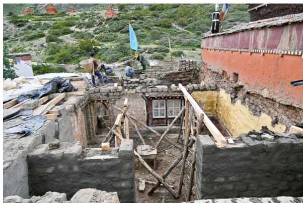
Figure 97: View of the back guest room after dismantling the roof. Note the new walls in the foreground.
