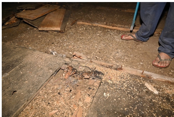
Figure 52: The dismantling of the wooden floor in the sanctum revealed rotten areas.
