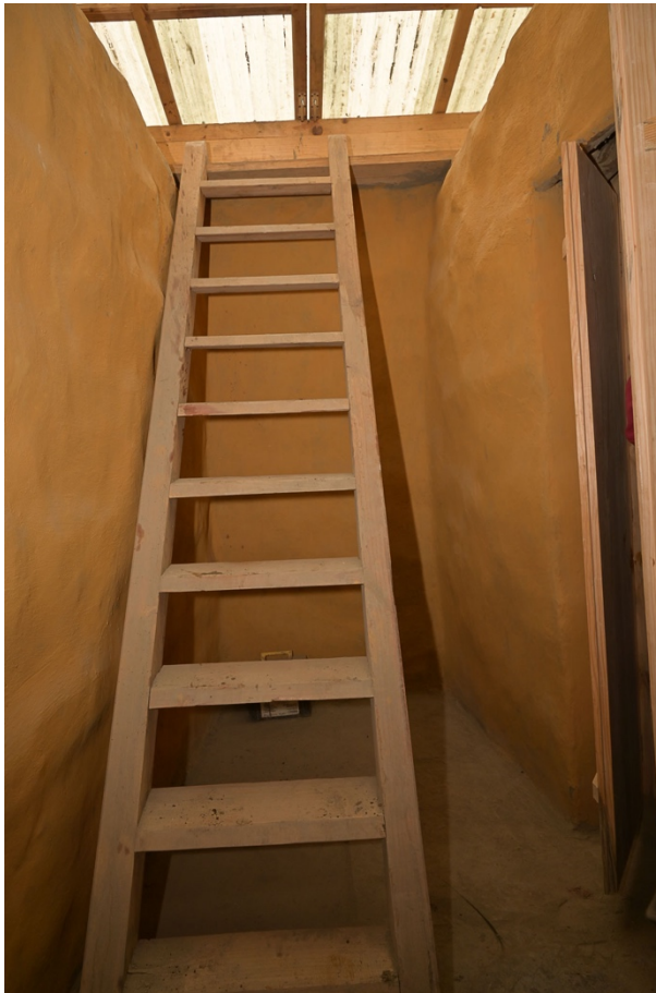
Figure 107: Roof access with its opening covered by a corrugated sheet skylight that can be opened.
