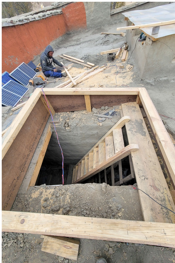
Figure 106: Roof access opening during construction.
