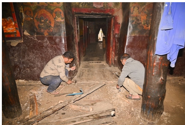
Figure 52: The dismantling of the wooden floor in the sanctum revealed rotten areas.
