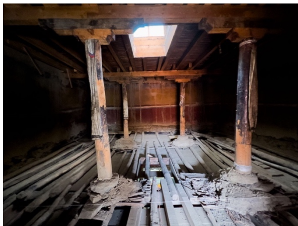
Figure 21: The Upper Sanctum with the mud floor removed. Note the uneven spacing of the joists and the precarious bases of the beams. The panelling underneath the joists are the false ceiling of the lower sanctum.
