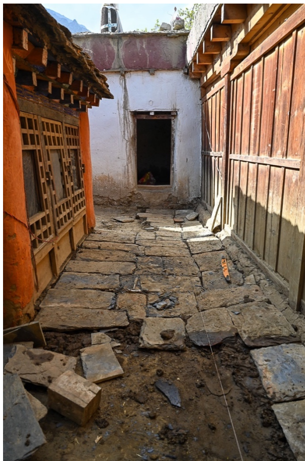
Figure 38: Paving the courtyard with stone. The door in the back leads to the new Arhat and Avalokiteśvara temples.
