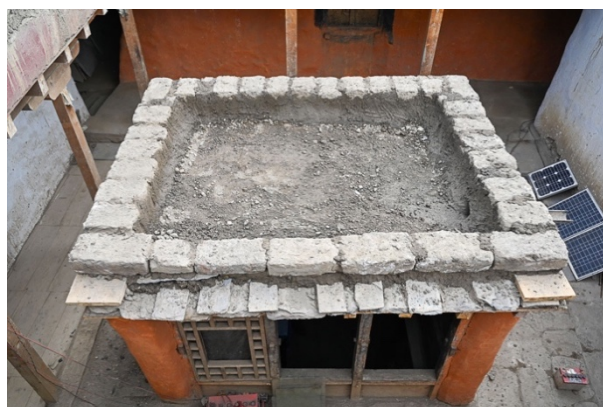
Figure 42: The lantern with the new roof and the lower parapet.
