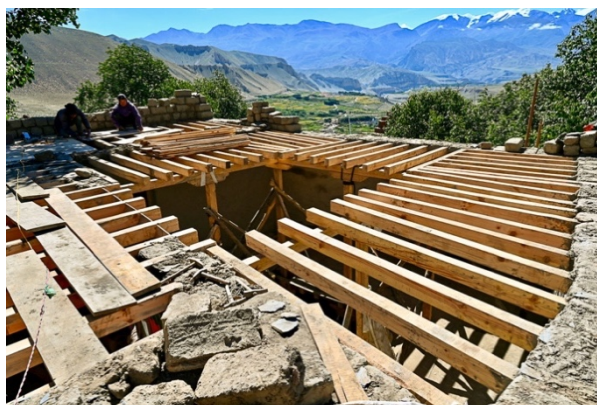
Figure 78: Reconstructing the timber structure of the atrium on the lower floor.
