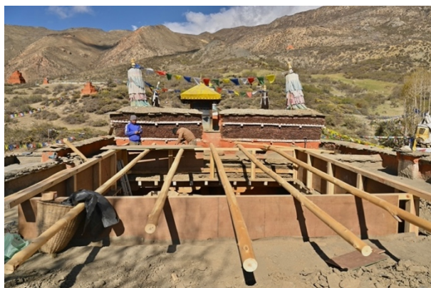
Figure 68: The construction of the frame for the roofing of the courtyard.
