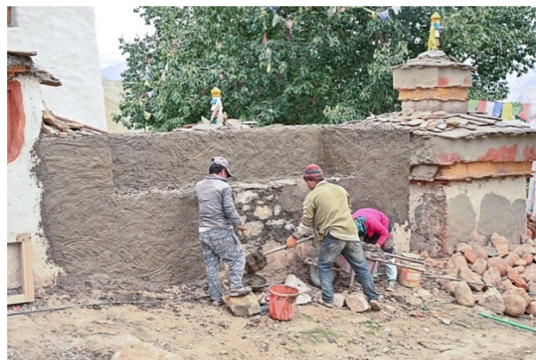
Figure 114: Uncovering the existing platform to build encasing for the prayer wheels.
