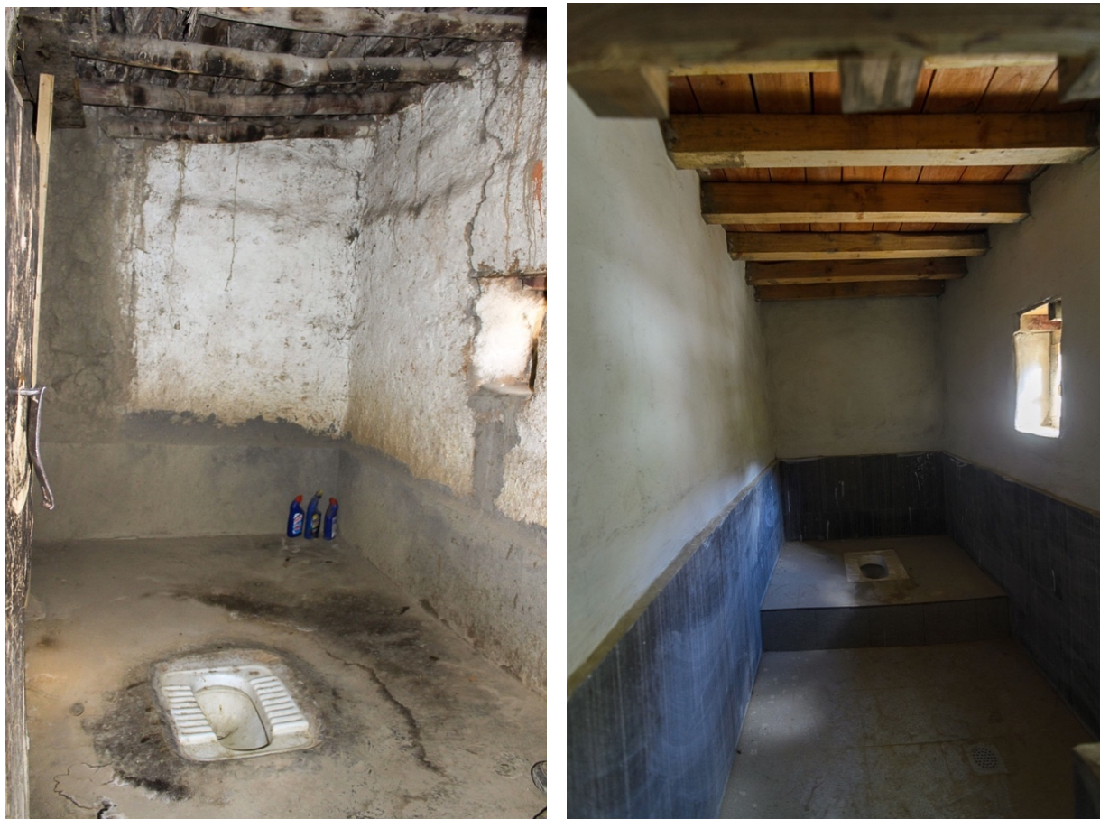
Figure 103: The toilet before and after restoration.
