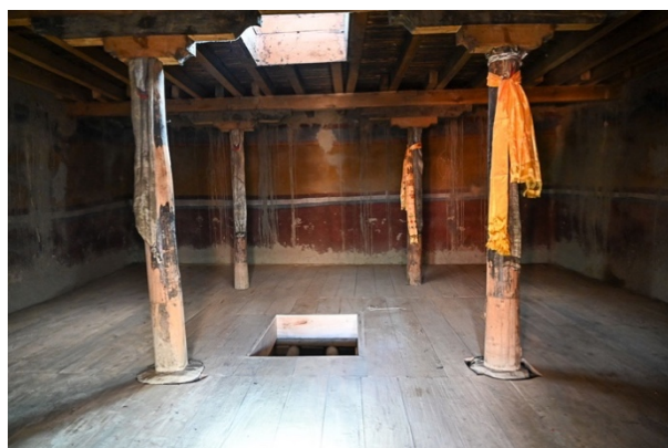
Figure 26: The Upper Sanctum with its new flooring completed.
