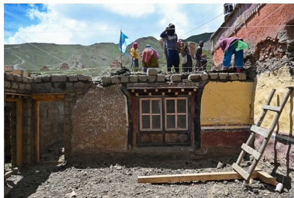
Figure 97: View of the back guest room after dismantling the roof. Note the new walls in the foreground.
