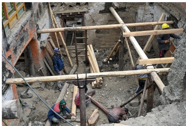
Figure 77: Reconstruction of the timber structure in the atrium after lowering its floor level.
