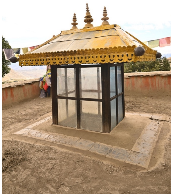
Figure 66: The previous tin sheet lantern room painted in yellow.
