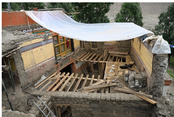
Figure 78: Reconstructing the timber structure of the atrium on the lower floor.
