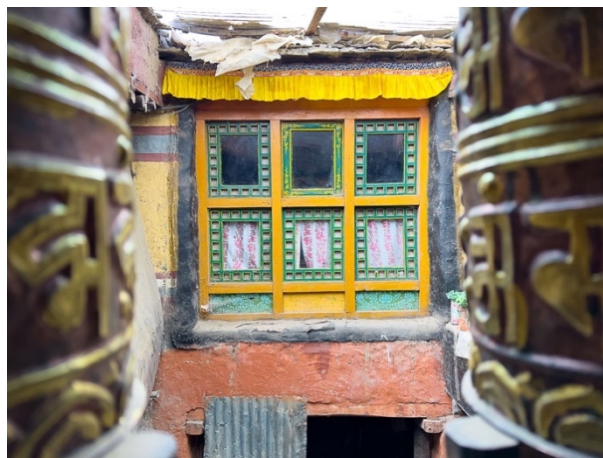
Figure 93: The window of the VIP room prior to restoration.
