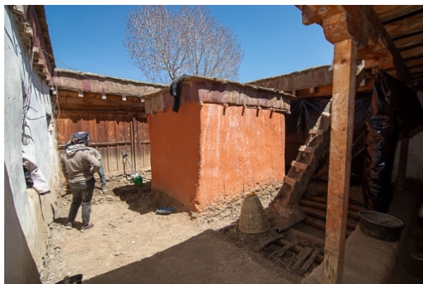
Figure 32: Removing of the mud floor in the courtyard.
