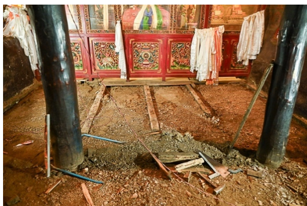
Figure 54: The previous floor of the sanctum removed.
