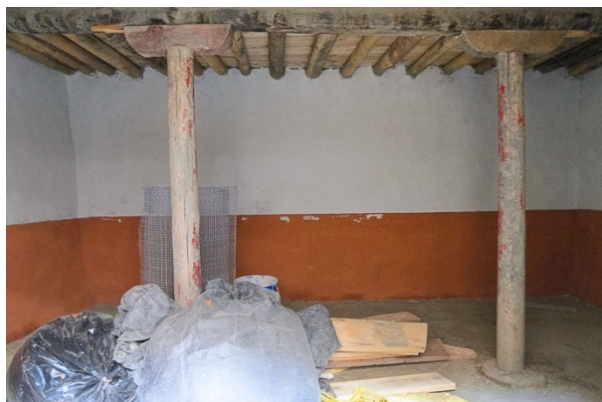
Figure 84: The storage room to the side of the atrium after restoration.
