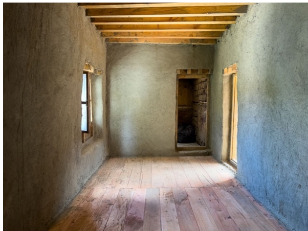
Figure 88: The new guestroom with attached bathroom during restoration.
