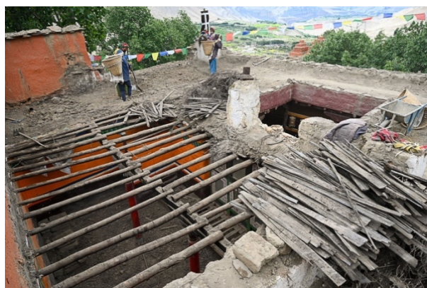
Figure 72: Removing the roof above the VIP room with the original joists exposed.
