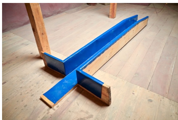
Figure 122: A new drainage spout ready for installation.
