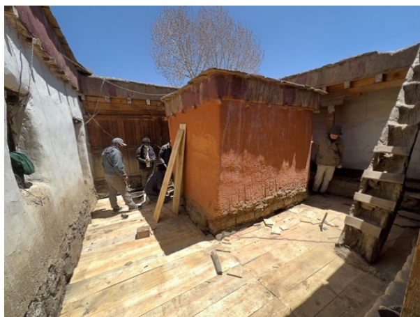
Figure 34: Planking on the original joists in the courtyard.
