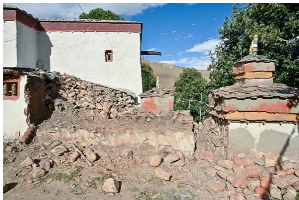
Figure 114: Uncovering the existing platform to build encasing for the prayer wheels.
