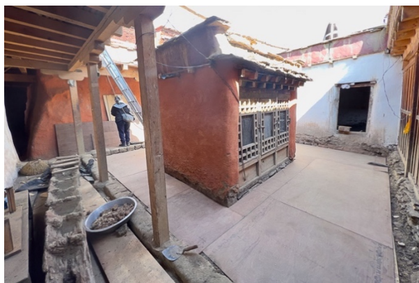
Figure 36: Waterproof plywood was attached to the wooden frame.
