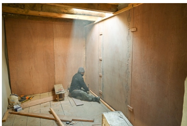
Figure 48: Construction of the double plywood shrine to hold the Avalokiteśvara stone panels.
