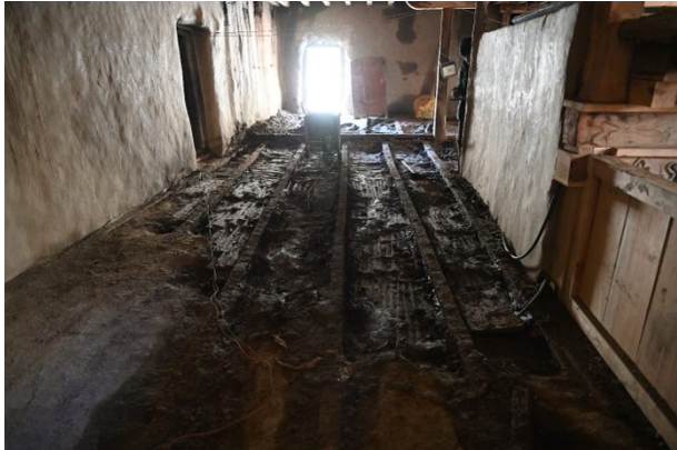
Figure 435: Parts of the floor on the upper level drenched in water after the rain.
