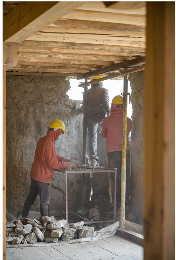
Figure 122: Supporting the cross beams of the northeast corner on the ground floor level.
