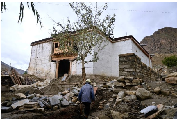
Figure 412: Photo taken on September after partially whitewashing the exterior walls.
