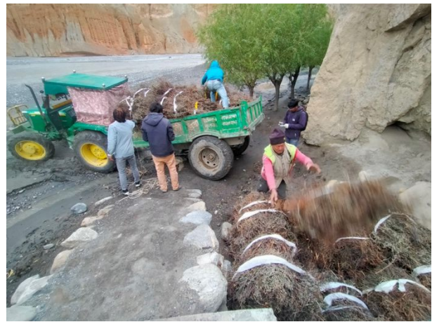
Figure 19: Weighing a bundle of dry grass purchased from the villagers to mix with mud for the adobe bricks.
