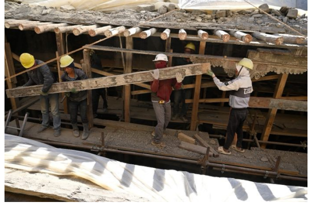
Figure 297: Dismantling the beams and long pillars along the third row that hold the superstructure above the painted wall.
