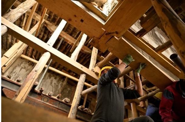
Figure 291: Placing the new plank underneath the reinstalled original beam.
