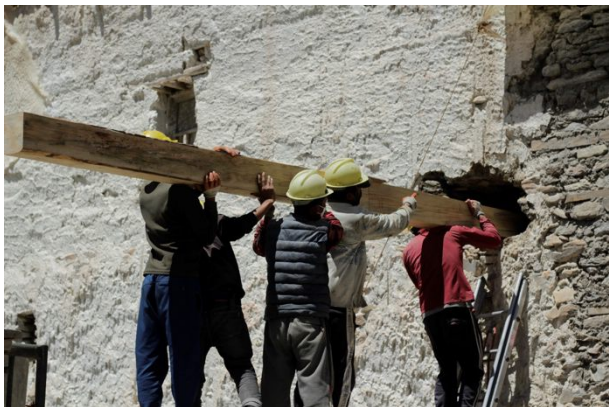
Figure 174: Inserting the new beam to replace old one through a hole in the south wall.
