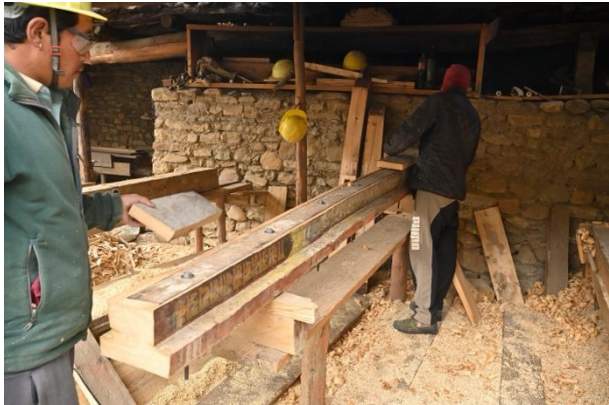
Figure 384: Restoration of the broken beam in the same manner as the one of the ground floor.
