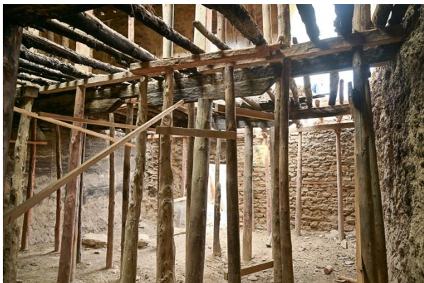
Figure 169: Installing temporary supports for the wooden members of the upper floor before dismantling.
