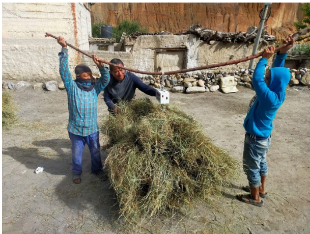
Figure 19: Weighing a bundle of dry grass purchased from the villagers to mix with mud for the adobe bricks.
