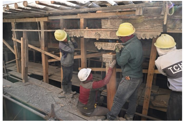
Figure 299: Preparing the repaired beams to be placed to their original position.
