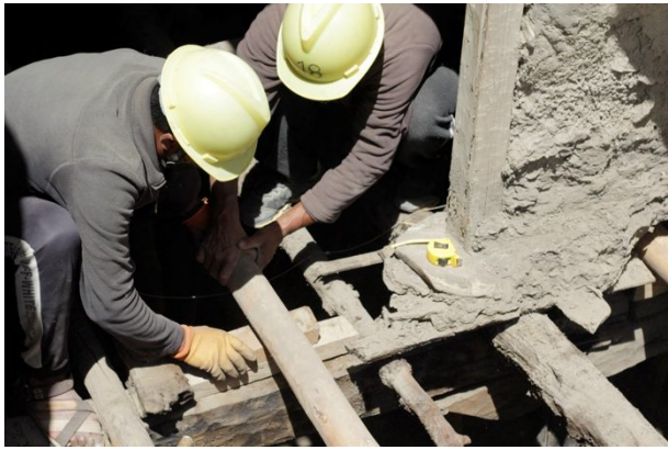
Figure 170: Replacing the old joist with new one maintaining the level.
