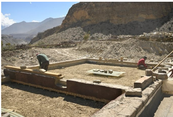
Figure 334: Laying the lower layer of mud on the roof of the South Wing.
