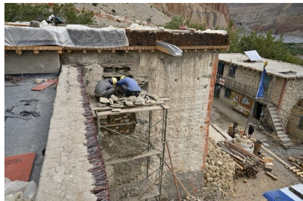
Figure 212: Repairing the lower floor corner of the Entry Hall with wooden ties.
