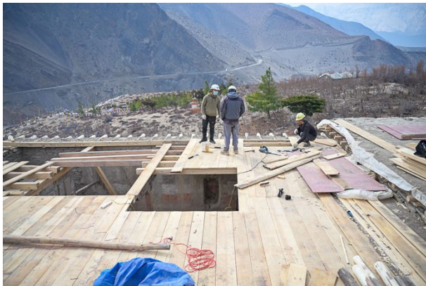
Figure 181: Adding the planking to the roof of the south wing.
