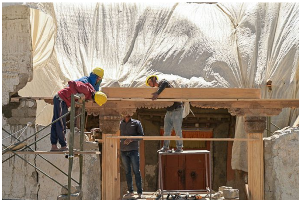
Figure 98: Arranging the positioning of the central beam as per measurements.
