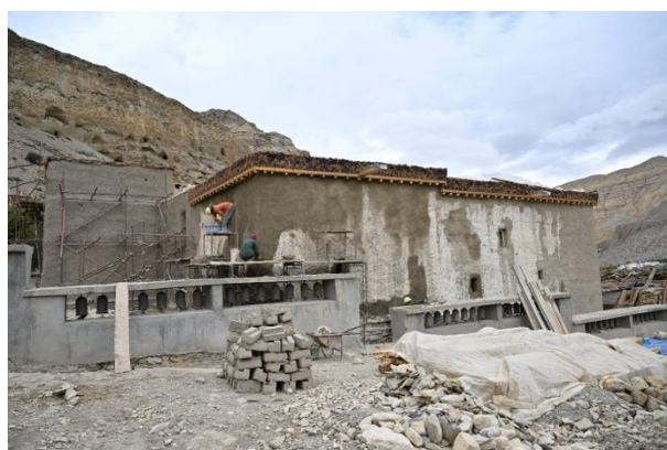
Figure 343: Plastering the exterior in the newly constructed corner of the South Wing.
