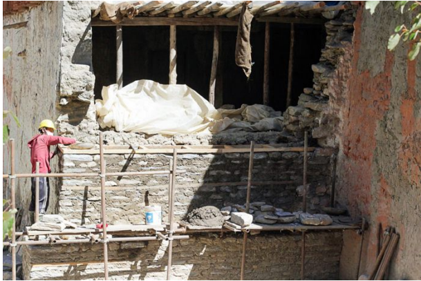
Figure 198: The wall reconstructed to the level of the first floor, where a wall-tie was inserted.
