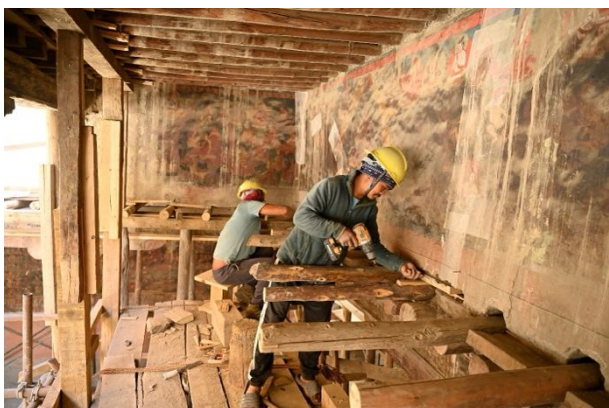
Figure 271: Inserting new joists into holes at a higher level of the painted wall.
