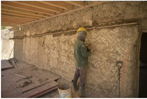
Figure 317: Preparing the wall above the entrance to the Assembly Hall for replastering.
