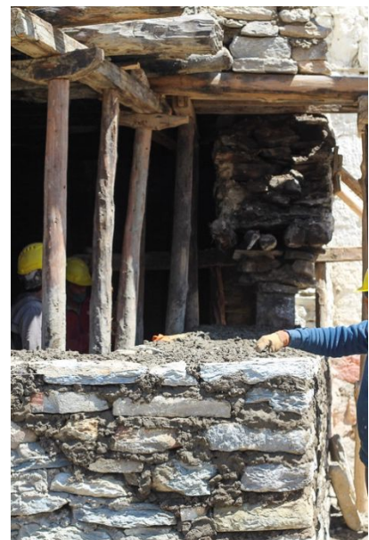
Figure 150: The east side of the corner with temporary supports added while preparing the foundation of the new wall.
