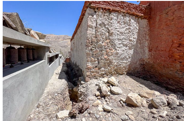
Figure 59: All along the outer wall of the monument a ditch was dug for the wall strengthening the foundation.
