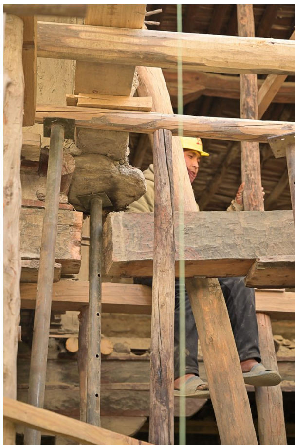
Figure 276: At this stage also the beam that supported the painted wall could be removed.
