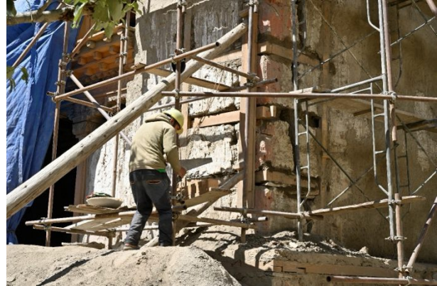
Figure 211: Repairing the large crack on the north wall of the Entry Hall with wooden ties.
