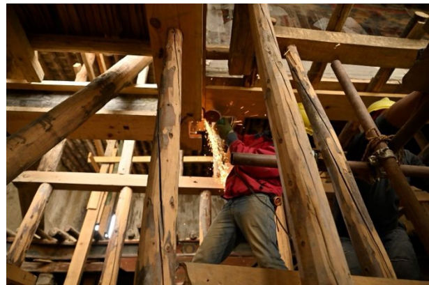
Figure 289: Preparing the placement of the restored beam underneath the painted wall.
