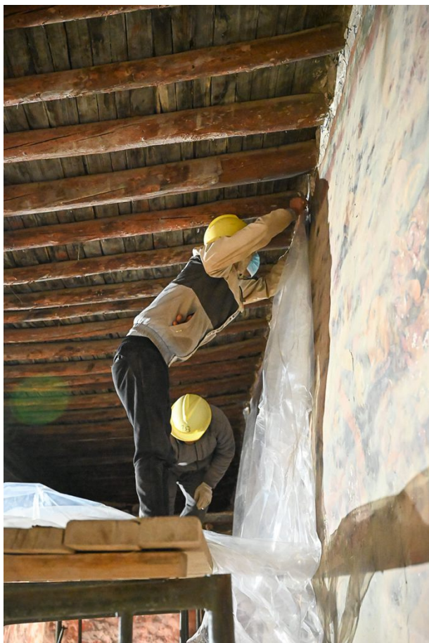
Figure 242: Attaching the plastic sheets to protect the murals of the Assembly Hall.
