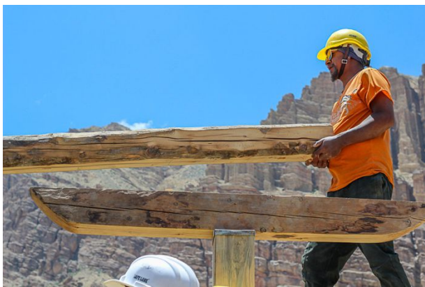
Figure 139: On the upper floor the old capitals could be retained while the pillars and a part of the beam had to be replaced. Note the joints between capital and beam for seismic strengthening.
