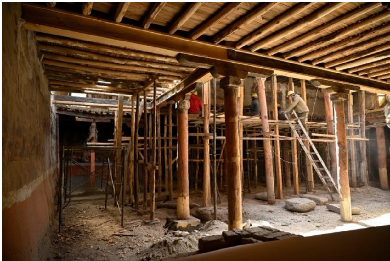
Figure 286: View from the restored section towards the fourth and fifth rows of pillars. On the right work commenced on replacing the support of the painted wall, while the broken beam in the last row and its support can be seen on the left.
