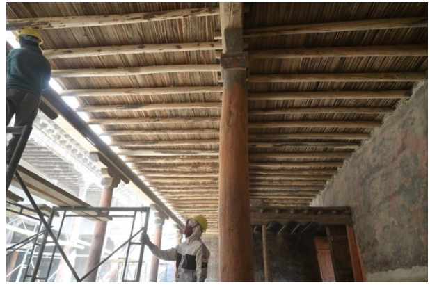
Figure 266: The first and second bay of the Assembly Hall after the reconstruction.
