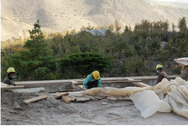
Figure 216: Installing the temporary roof above the south wing.
