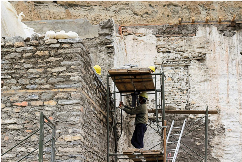
Figure 157: Continuing the construction of the southeast corner wall.
