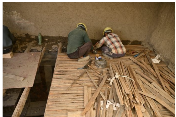
Figure 314: Replacing the rotten joists between row five and the back wall of the Assembly Hall. Note the Assembly Hall murals and the protective roof on the upper level.
