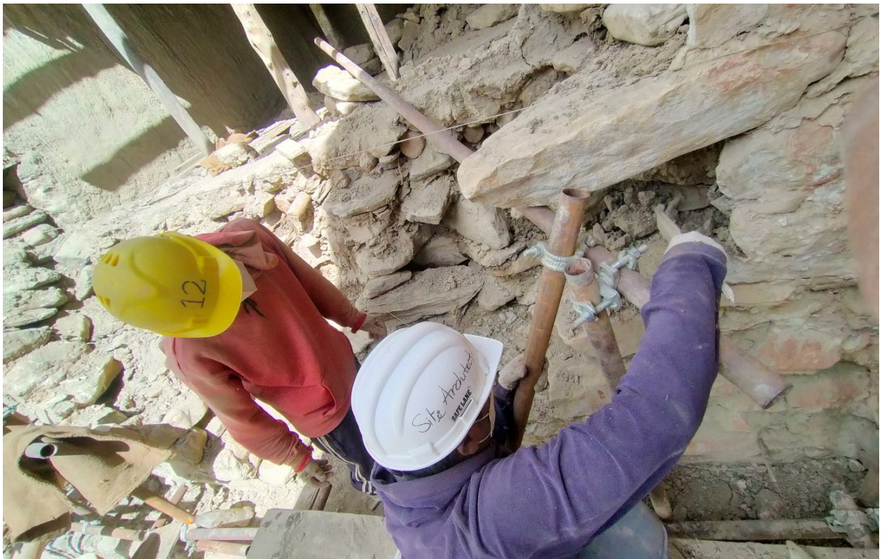
Figure 195: Supporting a large stone from the original wall that can act as connector between the old and new walls.
