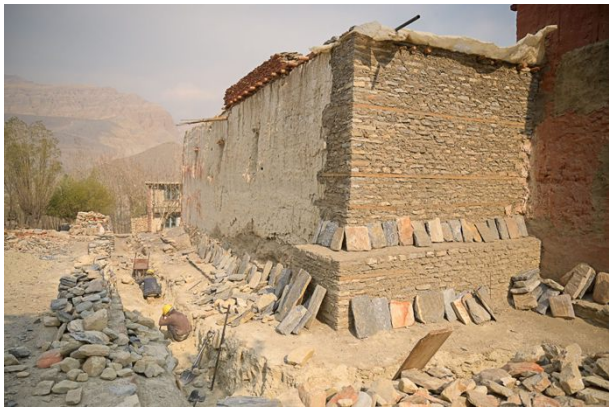
Figure 349: The northwest corner of the temple before plastering.
