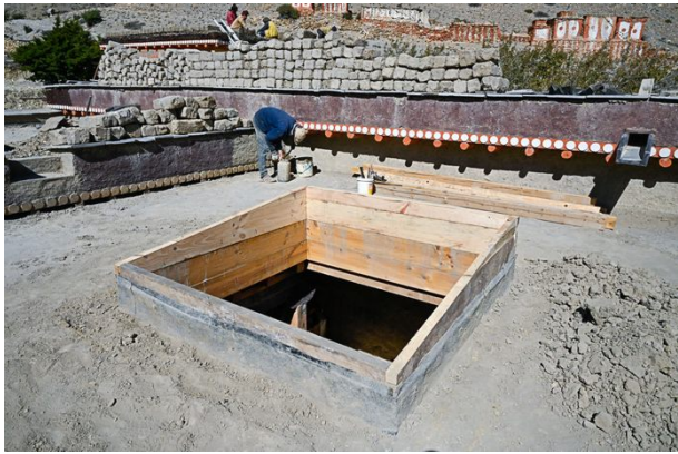
Figure 365: One of the skylights above the southern wing with its interior wooden frame.
