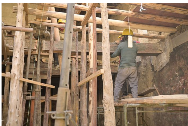
Figure 278: Removal of the beam on the wall side of the third row three on May 14.
