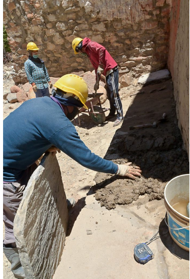
Figure 64: Covering the foundation support wall and the ground in front of it with mud.
