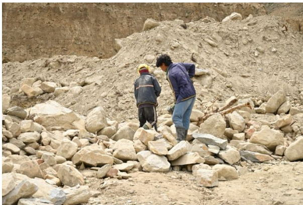
Figure 57: Sourcing and preparing local stone for the drainage and mani wall.
