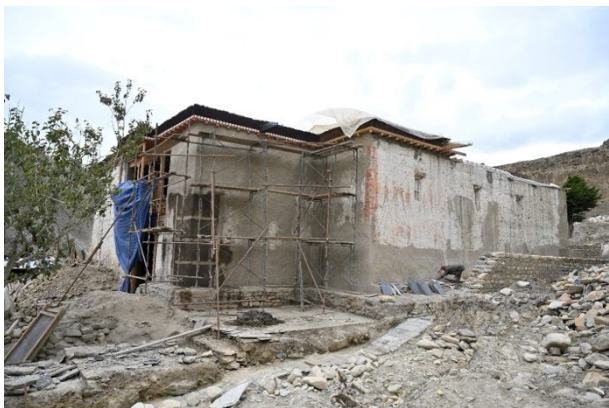
Figure 213: The repaired northeast corner of the Entry Hall after plastering.
