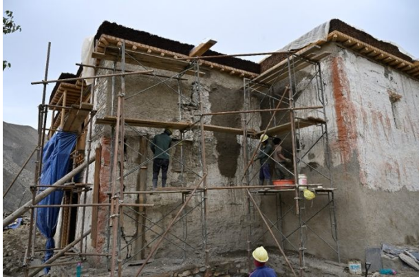
Figure 211: Repairing the large crack on the north wall of the Entry Hall with wooden ties.
