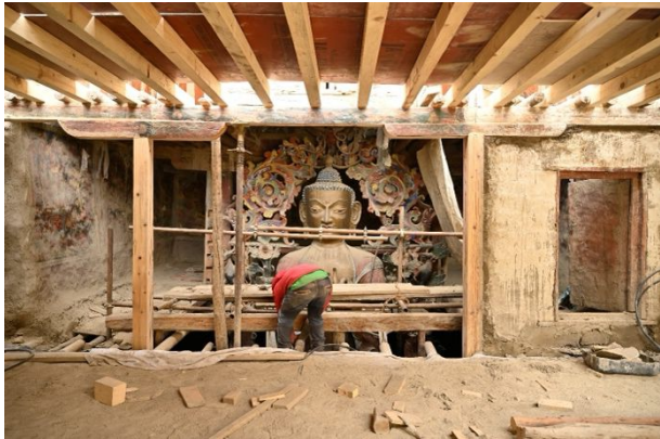
Figure 374: The upper-level area in front of the main sculpture after the main beam has been restored.
