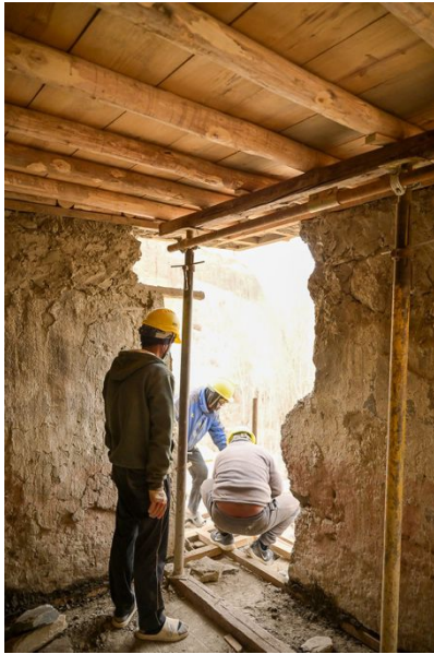
Figure 125: Placing the lowest wall tie on the upper floor of the northeast corner.
