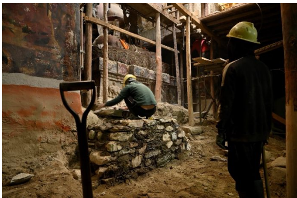
Figure 397: Construction of the staircase in front of the circumambulation path around the main image.
