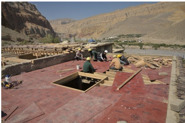
Figure 328: Constructing the wooden frame around the skylight.
