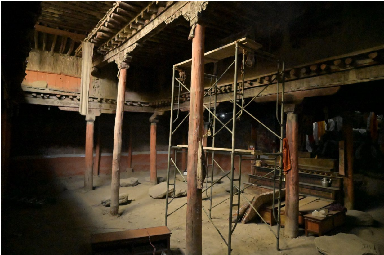
Figure 232: A scaffolding was set up to enable the measuring of the details of the large pillars.
