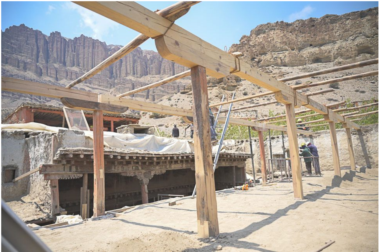
Figure 267: Reconstructing the upper level of the second row on May 2.
