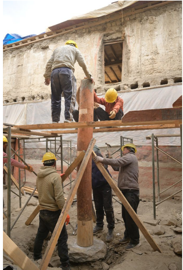
Figure 254: To ensure structural stability joints were created between each part of the capitals.
