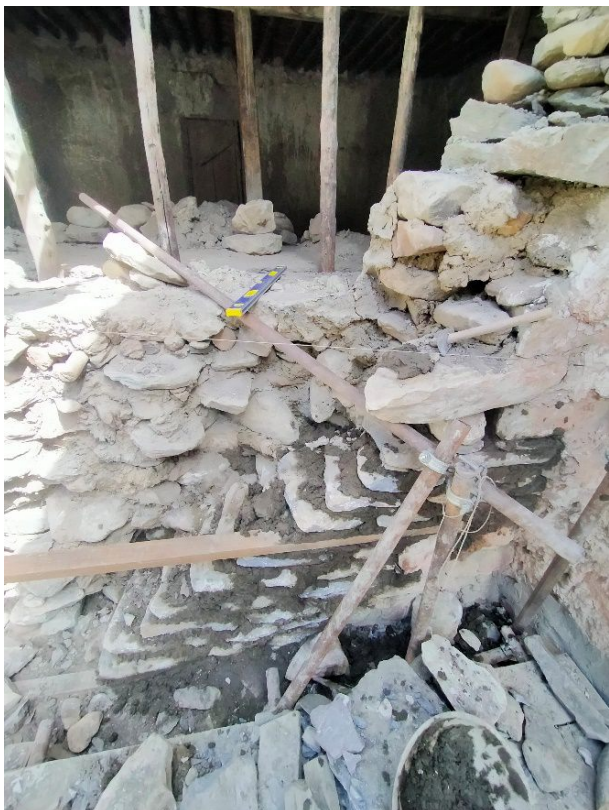
Figure 196: Construction of the new wall along the lower section of the wall and connecting it with the old one.
