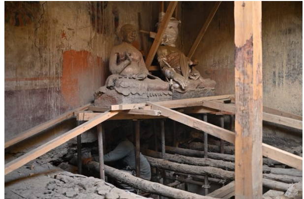
Figure 185: Installing supports from the sides to keep the sculptures in place.
