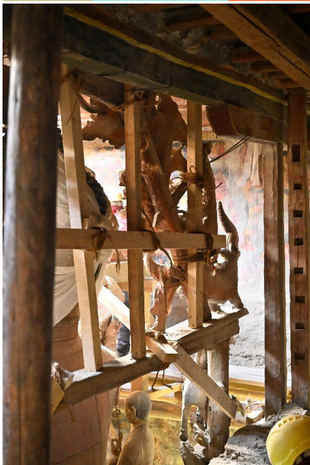
Figure 380: The support structure to the back of the main image.
