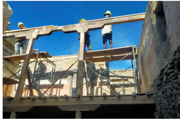
Figure 176: The ground floor level with half of the wooden structure already replaced.
