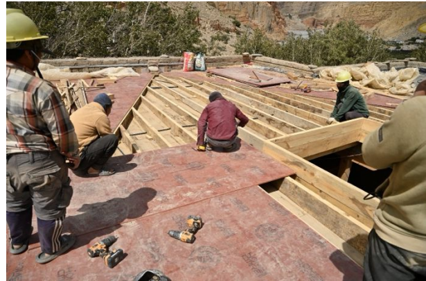
Figure 360: Once the planking was completed a frame to support the plywood at an angle was constructed.
