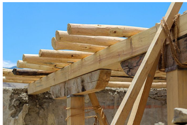
Figure 139: On the upper floor the old capitals could be retained while the pillars and a part of the beam had to be replaced. Note the joints between capital and beam for seismic strengthening.
