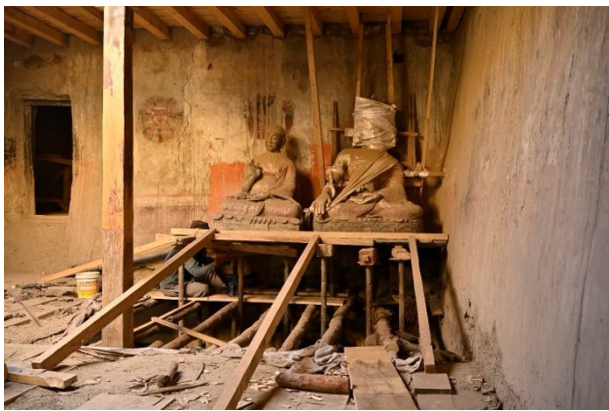
Figure 187: The supporting structure during the installation of the new joists.
