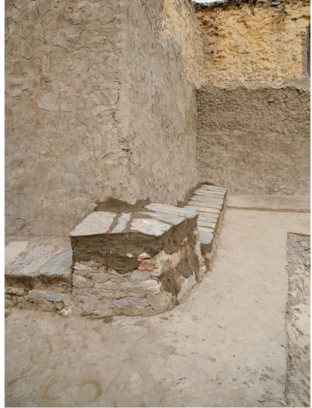
Figure 67: Mud was also laid between the newly constructed foundation support and the drainage.
