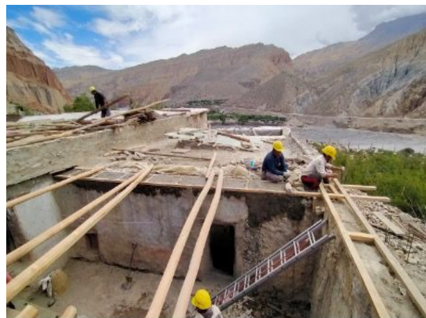
Figure 141: The structural wooden members for the roofing of the southwestern room prepared for assemblage.
