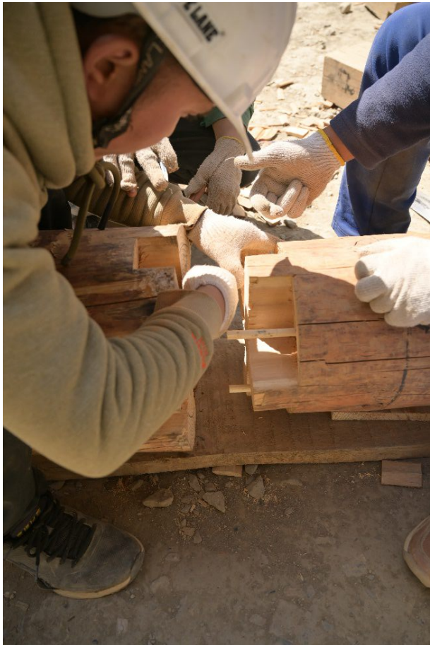
Figure 250: Once the structure was taken down the rotten bottom parts of the pillars were replaced.
