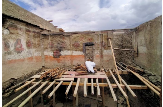
Figure 174: Inserting the new beam to replace old one through a hole in the south wall.
