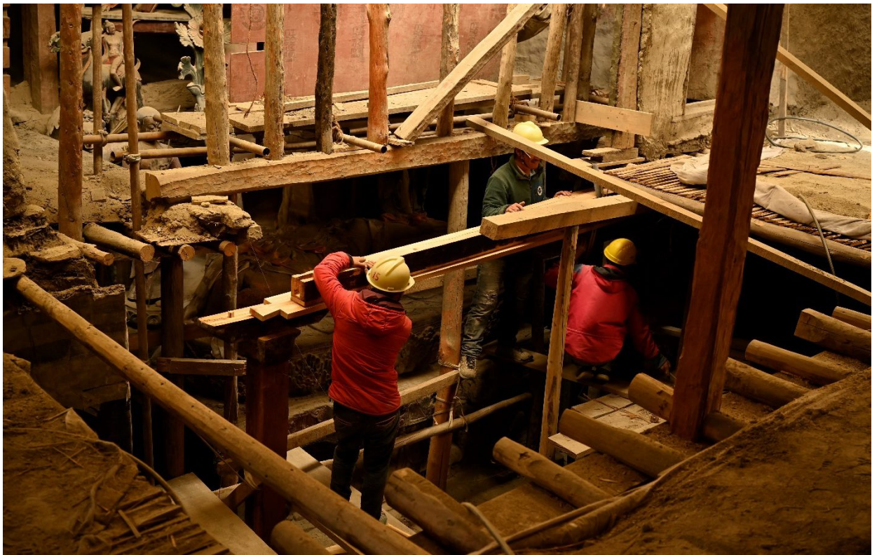
Figure 371: Reassembling the beam in front of the main sculpture after restoration; note the joints.
