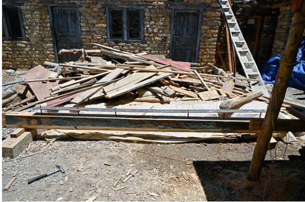
Figure 312: Placing iron plates on both sides of the broken beam.
