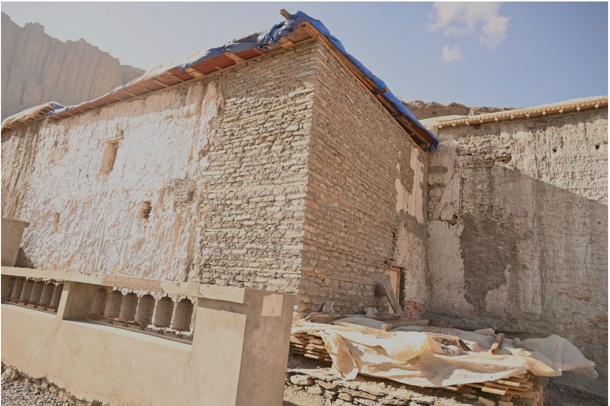
Figure 218: The temporary roof after completion late in 2023.
