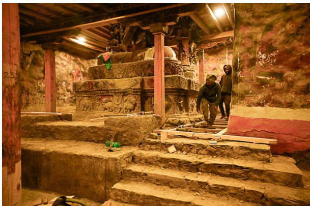
Figure 415: Installing the wooden frames for flooring the Ambulatory around the Maitreya sculpture. Note the massive flight of stairs installed at that stage.
