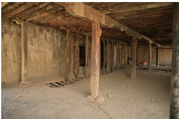
Figure 284: Preparation of the restoration of rows four and five by installing additional supports.
