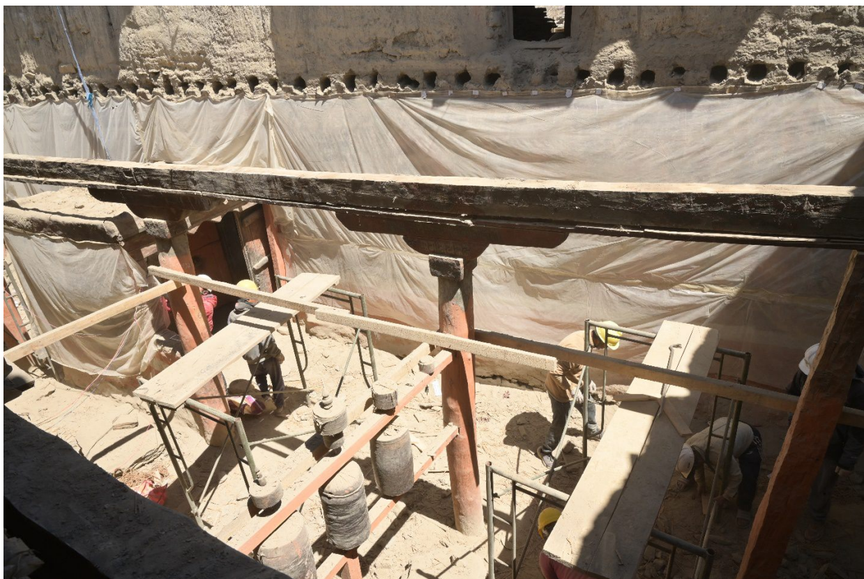
Figure 247: View into the entry area of the Assembly Hall after the dismantling of the level above it.
