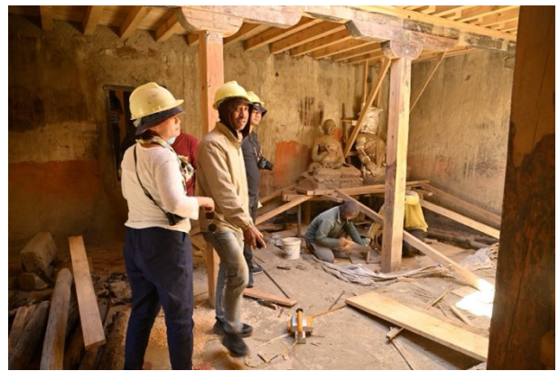
Figure 187: The supporting structure during the installation of the new joists.
