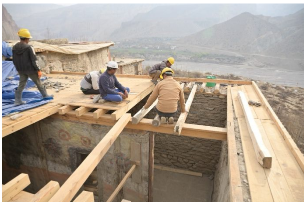
Figure 324: Finishing the roof above the painted room of the South Wing.
