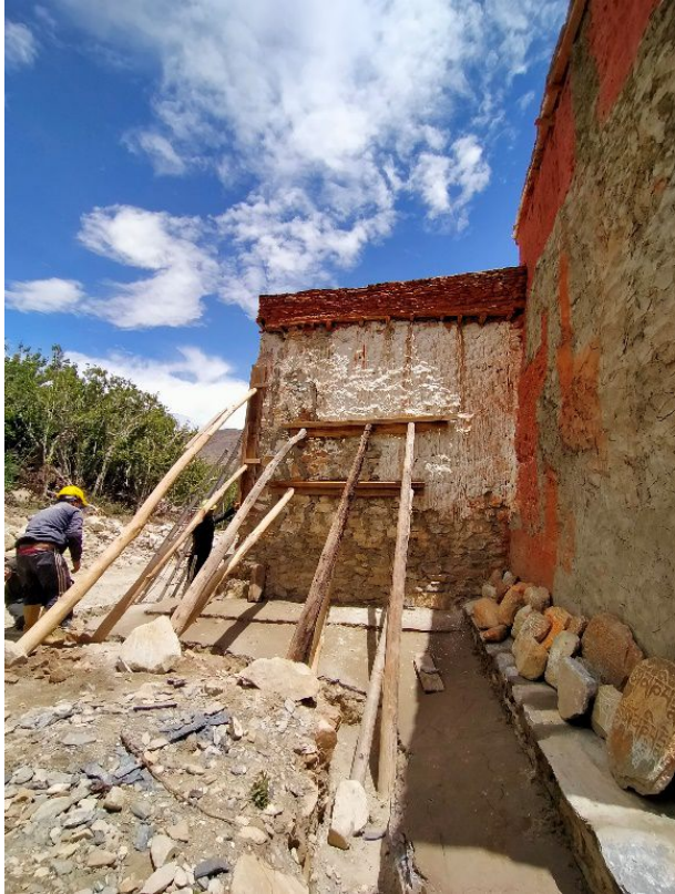
Figure 191: First the wall was shored up to prepare the dismantling from the top.
