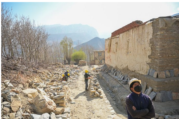
Figure 49: Preparation of the stones and the drainage canal on the north side of the temple.
