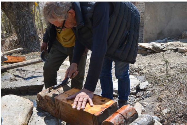
Figure 83: All original wooden members were cleaned and prepared for reconstruction, as demonstrated by Thomas Schrom here.
