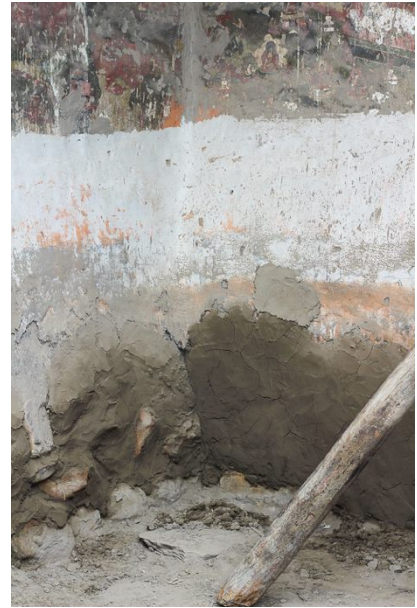
Figure 205: In this section on the west side of the monument plaster needed to be applied between the stones.
