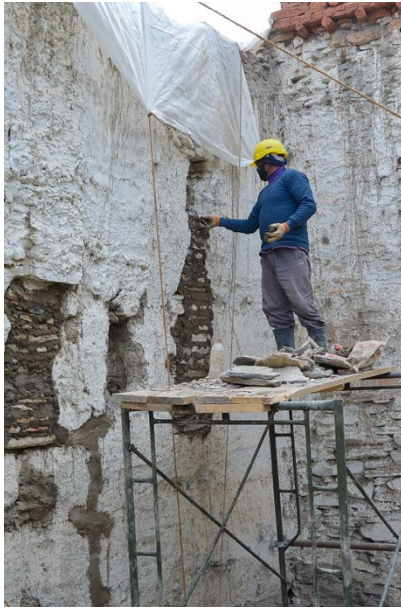
Figure 204: Here an area of loose stones was relayed.
