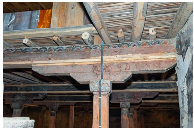
Figure 458: View of the distortion of the wooden structure due to the sagging of a pillar immediately in front of the main Buddha image.
