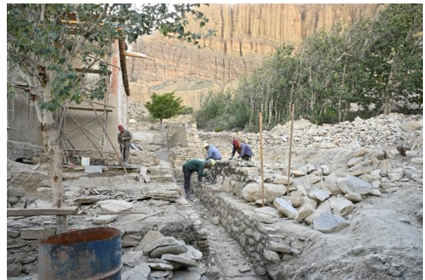
Figure 57: Sourcing and preparing local stone for the drainage and mani wall.
