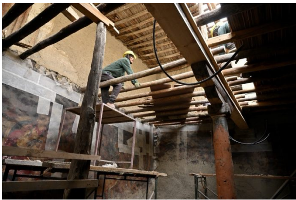
Figure 314: Replacing the rotten joists between row five and the back wall of the Assembly Hall. Note the Assembly Hall murals and the protective roof on the upper level.
