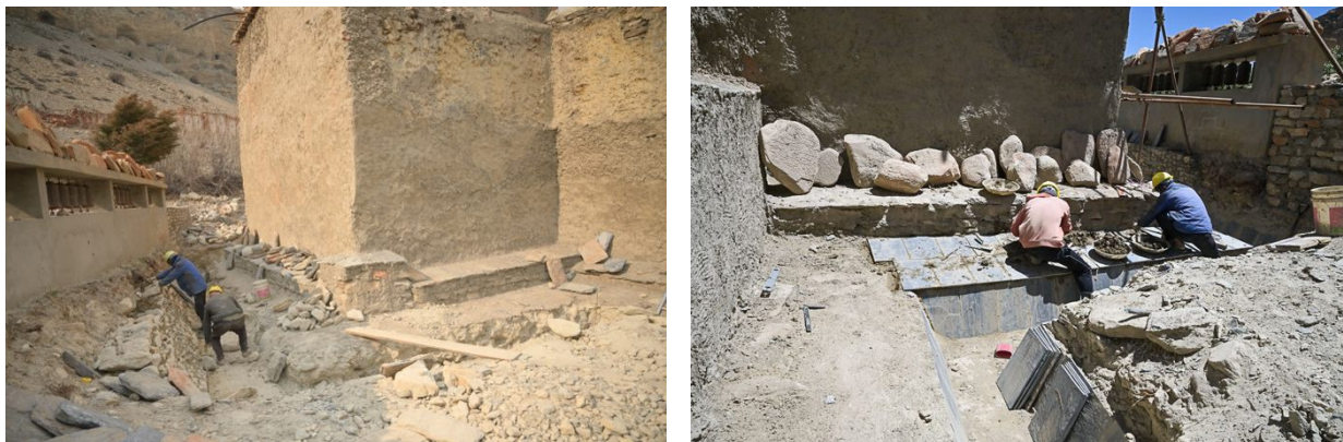
Figure 51: Making the stone wall for the drainage at the back of the temple.
