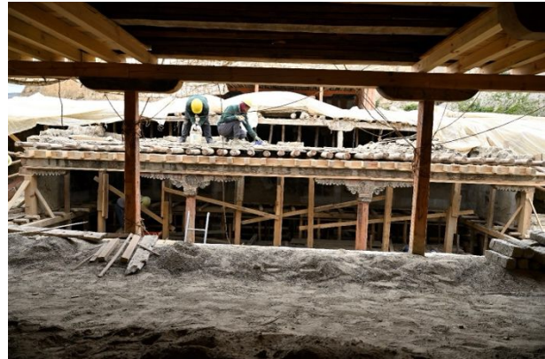
Figure 303: Rebuilding the structure above the reassembled beam following the original construction.
