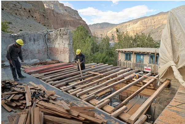
Figure 100: Arranging the original joist of the Entry Hall.
