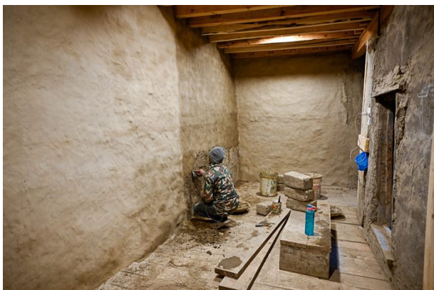
Figure 408: Fine plaster was applied to all the undecorated walls of the upper floor.
