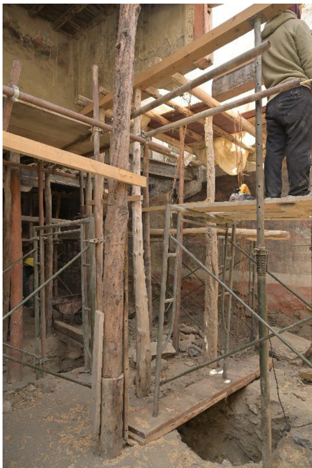
Figure 276: At this stage also the beam that supported the painted wall could be removed.
