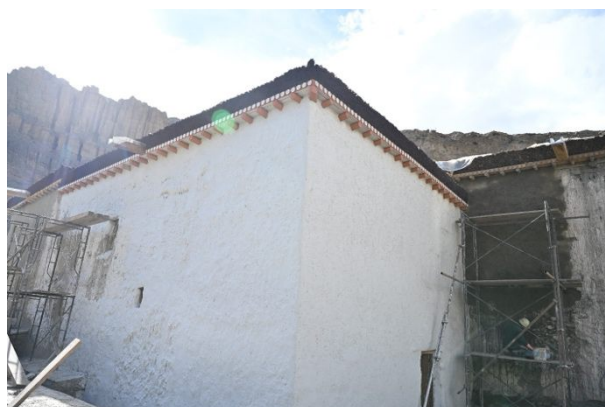
Figure 345: Repairing and plastering the southwest corner of the South Wing.
