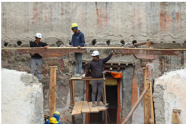
Figure 87: Once the two pillars were erected the laying of the beams was prepared by first placing the boards.
