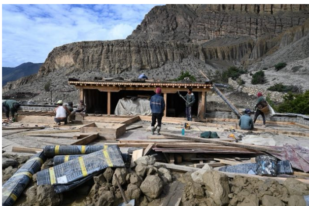
Figure 394: The wooden structure of the roof of the third level completed.
