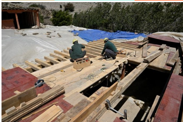
Figure 355: Roof work around the skylight.
