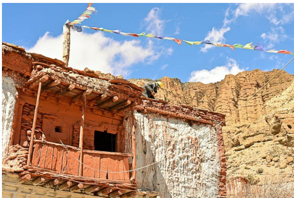
Figure 75: Dismantling of the porch area started from roof.
