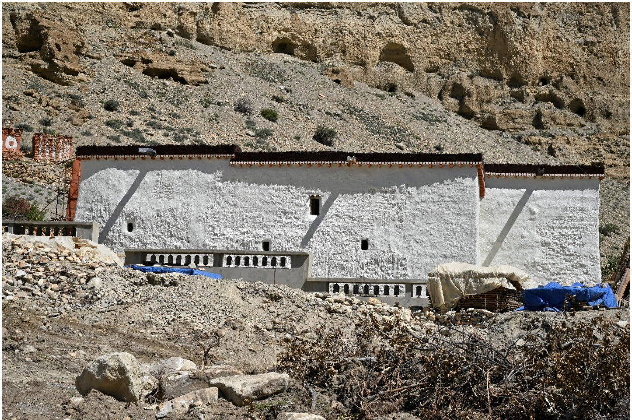
Figure 348: The South Wing after completing the painting work.
