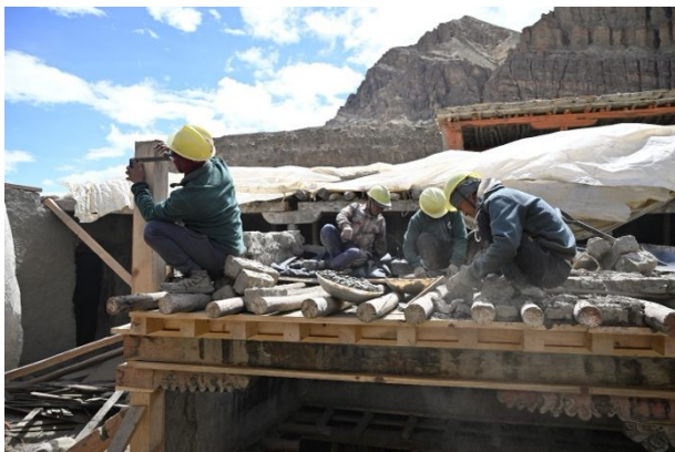
Figure 305: Realigning the joists and placing the corner pillar to support the roof above the painted wall area.
