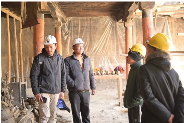
Figure 239: Inspection of the work on site.
