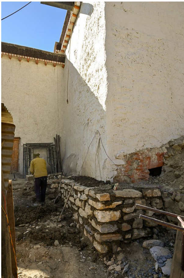
Figure 426: Expanding the foundation support around the southeast corner of the Entry Hall.
