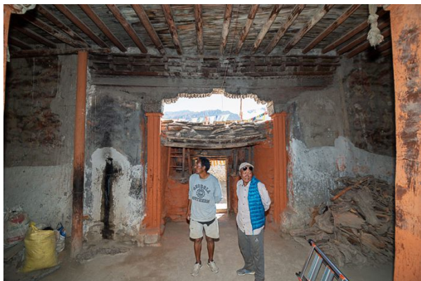
Figure 445: View of the entrance before restoration.
