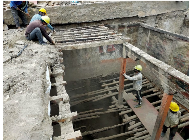
Figure 167: View of the painted room after removing its floor to enable the replacement of the wooden structure underneath.
