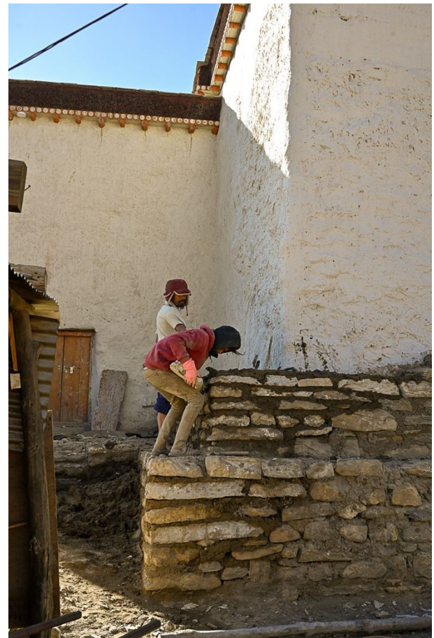
Figure 426: Expanding the foundation support around the southeast corner of the Entry Hall.
