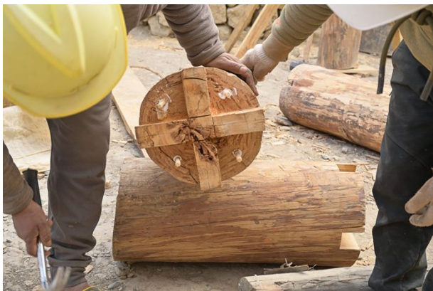
Figure 252: View of the cross shaped joint used to connect the old and new parts of the pillar.
