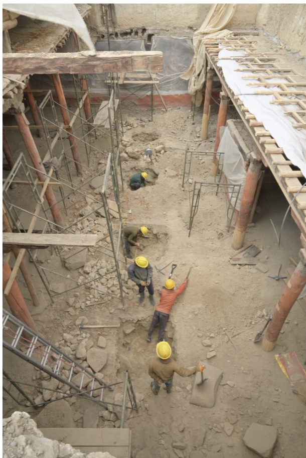
Figure 261: Preparing the foundation for the pillars of the second row.
