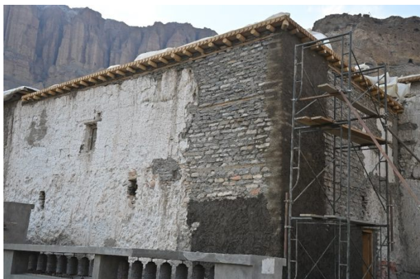
Figure 343: Plastering the exterior in the newly constructed corner of the South Wing.
