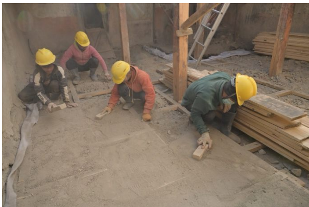
Figure 338: Filling the areas between the wooden frame with mud.
