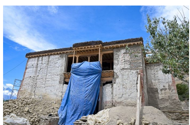
Figure 353: Parapet with Perma and waterspouts installed on the entrance side of the temple.
