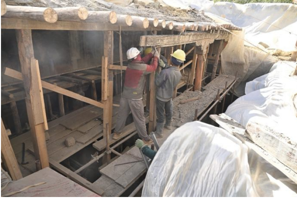
Figure 297: Dismantling the beams and long pillars along the third row that hold the superstructure above the painted wall.
