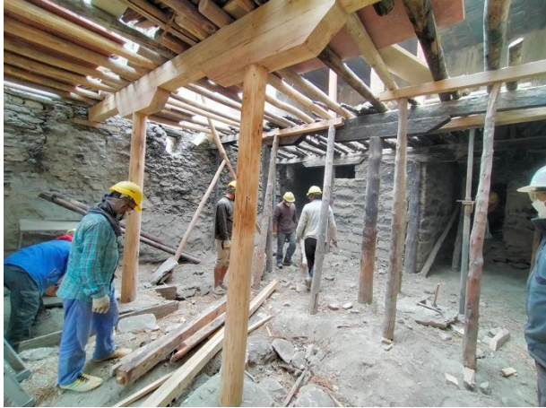
Figure 176: The ground floor level with half of the wooden structure already replaced.
