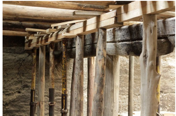
Figure 173: Supports were installed to preserve the painted partition wall above during reconstruction.
