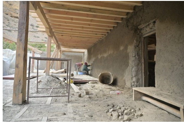
Figure 317: Preparing the wall above the entrance to the Assembly Hall for replastering.
