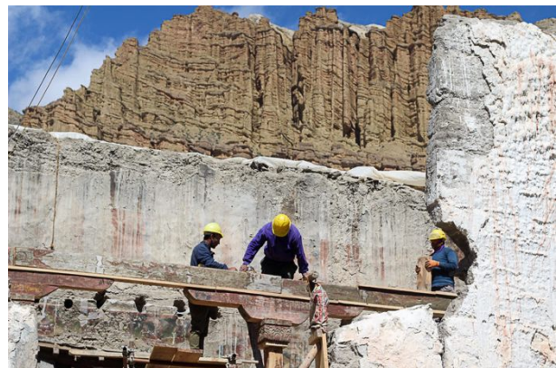
Figure 87: Once the two pillars were erected the laying of the beams was prepared by first placing the boards.
