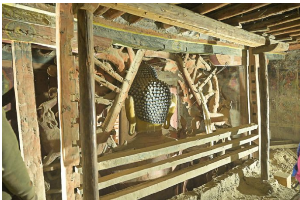
Figure 376: Removal of the frame behind the main image's head to expose the broken beam in this area.
