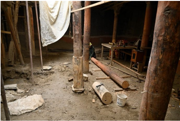
Figure 299: Preparing the repaired beams to be placed to their original position.
