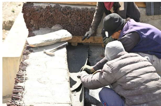
Figure 330: Construction of the traditional parapet with the apple twig bundles on the outside.
