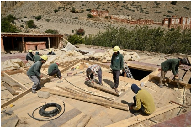
Figure 360: Once the planking was completed a frame to support the plywood at an angle was constructed.
