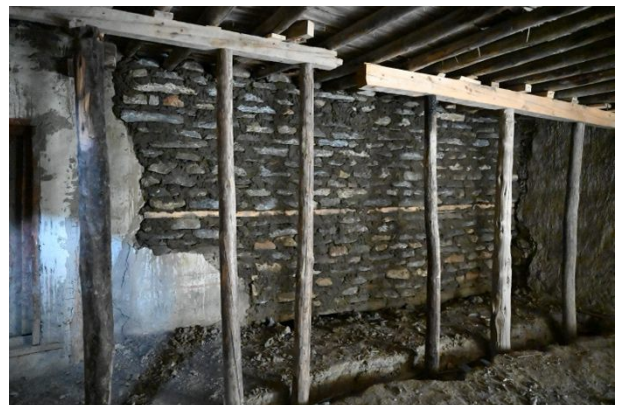
Figure 200: Installing the temporary roof above the new northwest corner wall.
