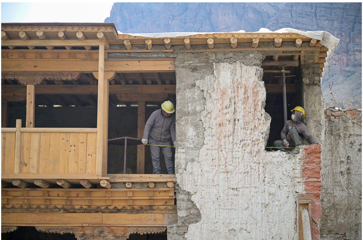
Figure 124: The upper part of the northeast corner after dismantling.
