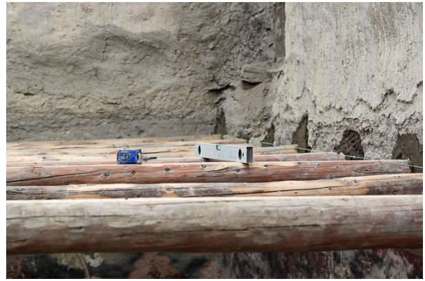
Figure 89: On the wall sides the reassembled beam was placed on a leveled stone plate inside the wall.
