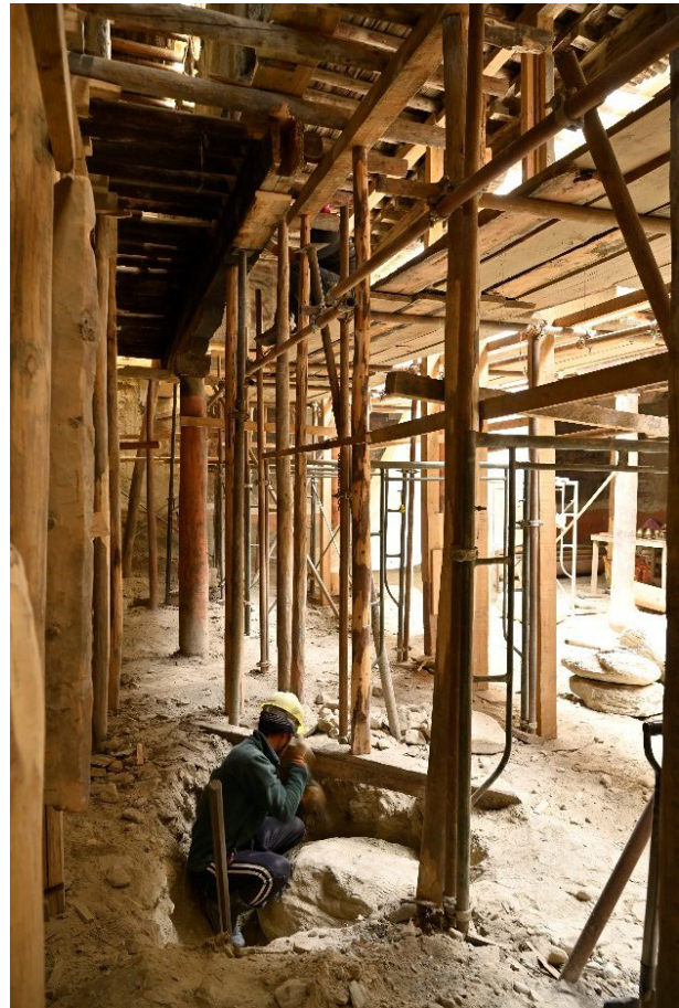
Figure 287: The temporary support structure underneath the painted wall with the original pillars removed.
