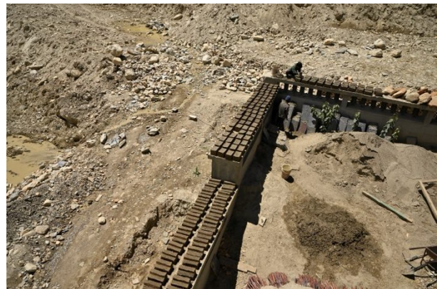
Figure 25: Preparing the mud mixture with hay and straw for the mud-bricks and rough plaster.
