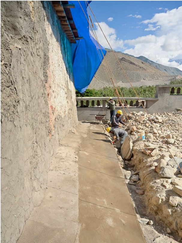
Figure 67: Mud was also laid between the newly constructed foundation support and the drainage.
