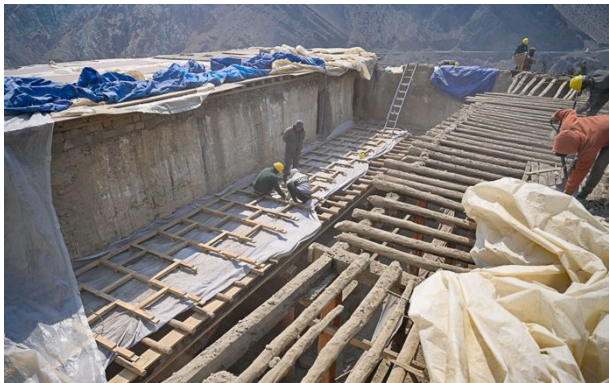
Figure 259: Creation of floor frame for the first bay while the roof above the third bay is being dismantled on April 11.
