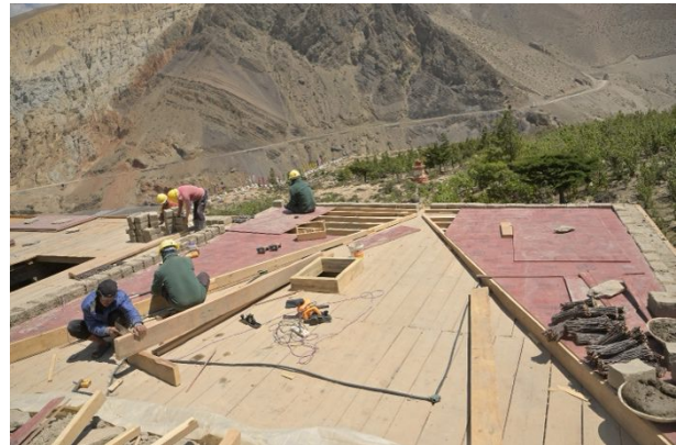
Figure 326: Constructing the wooden frame for the plywood with the sloping.
