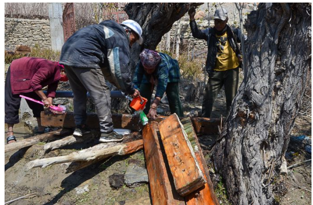
Figure 83: All original wooden members were cleaned and prepared for reconstruction, as demonstrated by Thomas Schrom here.
