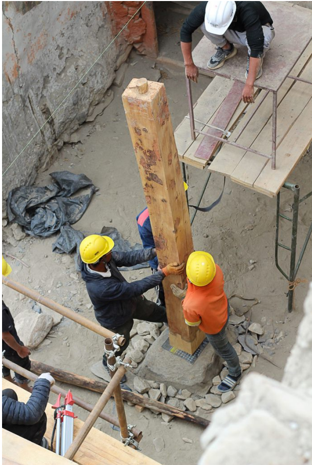
Figure 85: The original pillar, expanded in height, was joined with a new bedrock.
