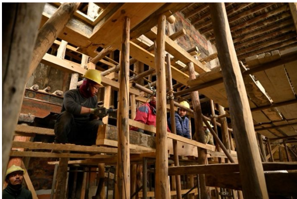
Figure 289: Preparing the placement of the restored beam underneath the painted wall.
