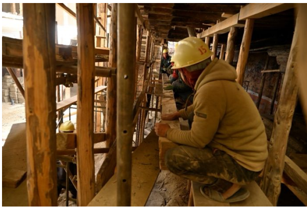
Figure 293: Workers ready to lift the second beam into its place underneath the painted wall.
