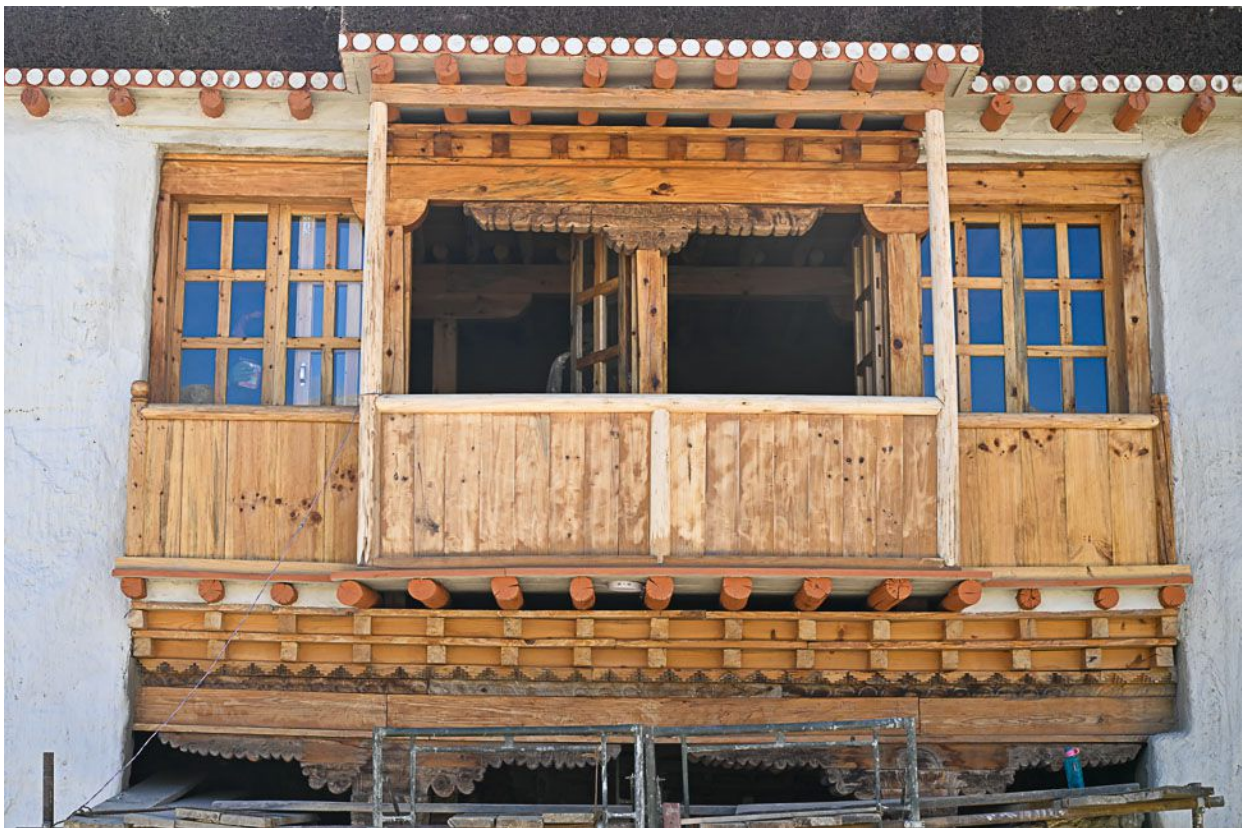
Figure 132: View of the balcony with the doors installed but opened in the central area. Note also the screens added at the sides to give the balcony a uniform appearance.
