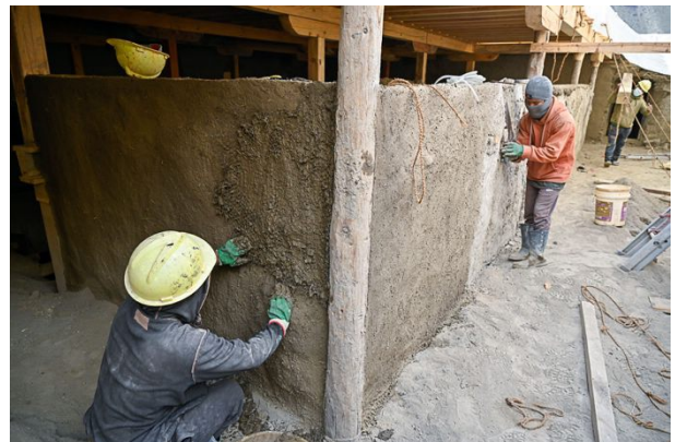
Figure 402: Application of the final mud plaster on the walls of the upper level.
