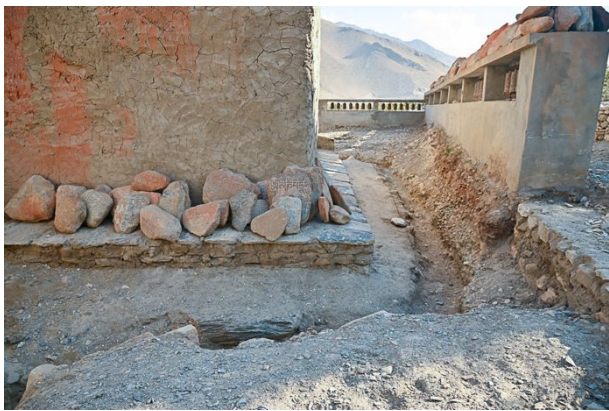
Figure 47: Foundation support and drainage at the back of the temple in October 2023.
