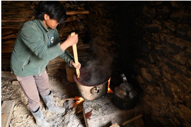
Figure 23: Preparing the maroon color for the parapet brushwood.
