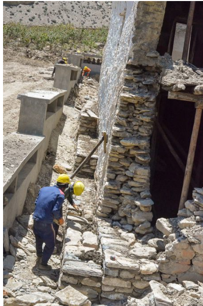
Figure 147: Supports needed to be installed in different areas of southeast corner.
