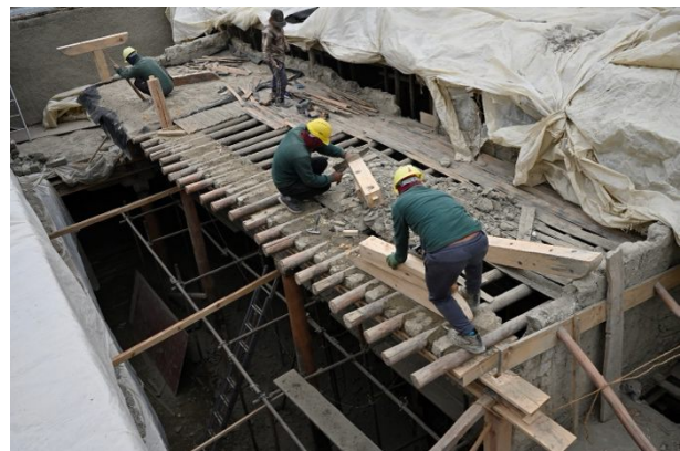
Figure 305: Realigning the joists and placing the corner pillar to support the roof above the painted wall area.
