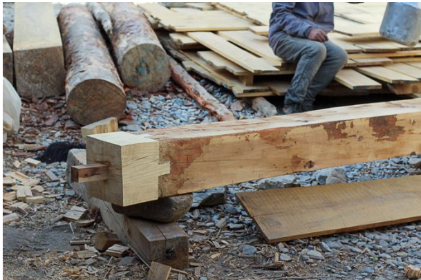
Figure 81: The original post holding the porch was lengthened by adding a new bottom section.
