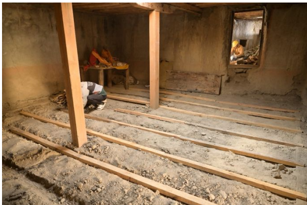
Figure 337: Preparing the frame for blanking in the South Wing rooms.
