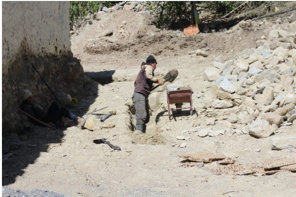
Figure 45: A worker digging the drainage channel at a distance to the temple's walls.
