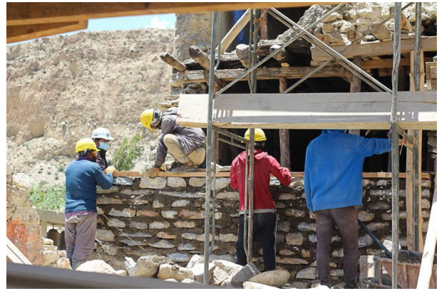
Figure 153: Wooden wall ties were added to the wall for seismic strengthening.
