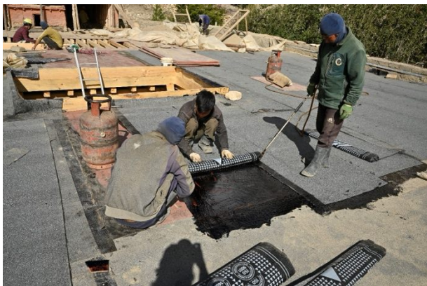
Figure 362: Installing bitumen sheets on top of the plywood.
