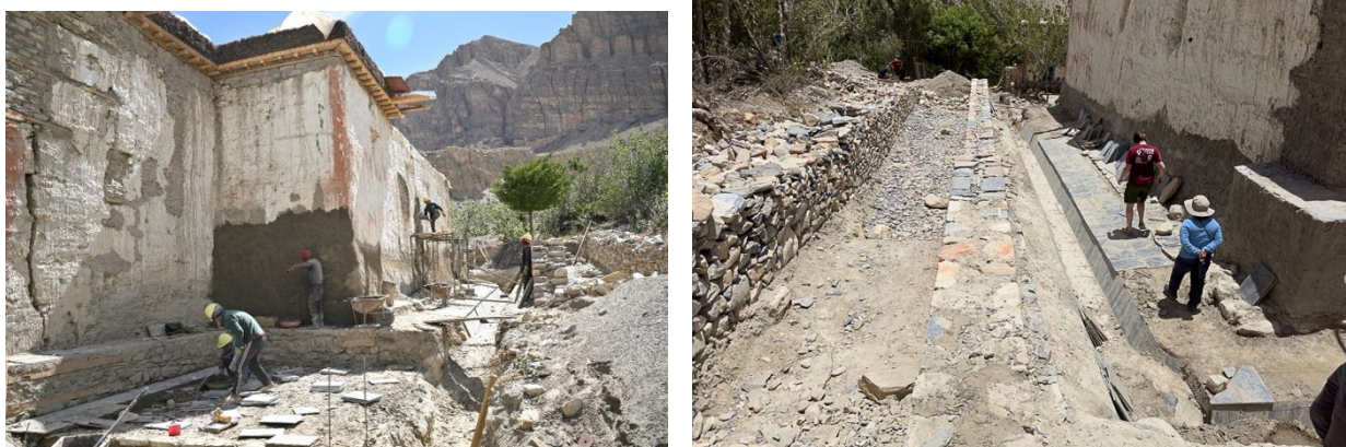
Figure 53: Works at the slope side of the temple including the installation of slates to ensure runoff towards the drainage.
