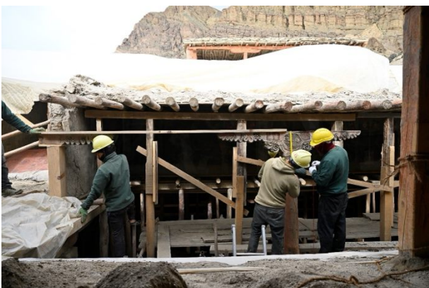
Figure 301: Continuing to reassemble the original structure supported by the long pillars.
