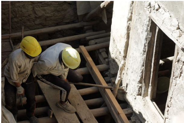
Figure 172: Placing another joist under the partition wall.
