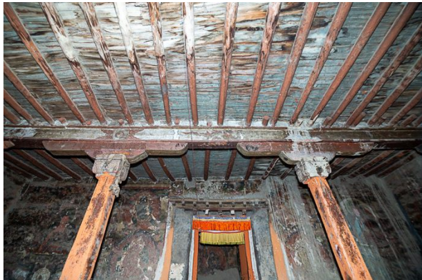
Figure 447: View of the west wall of the Entry Hall before restoration.
