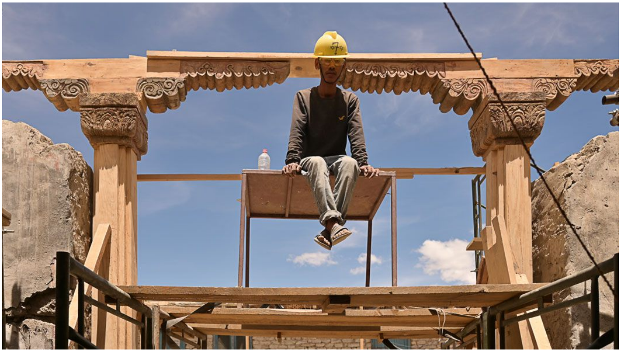
Figure 97: A worker taking a short rest during the reconstruction of the entry porch.
