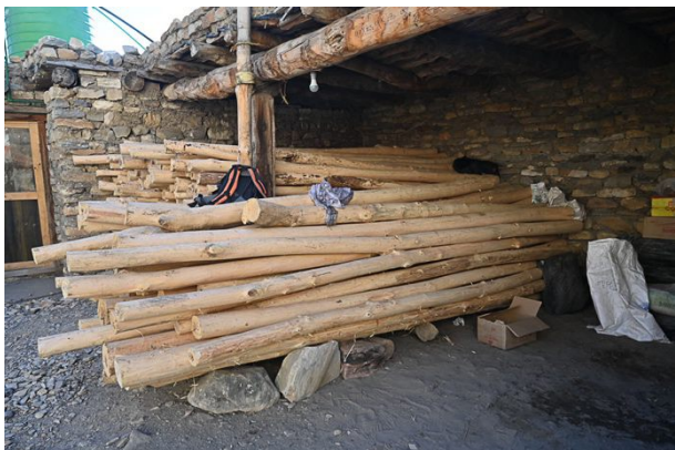
Figure 17: Poplar joists procured at Gyakar village stored at the site.
