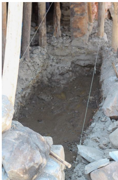
Figure 150: The east side of the corner with temporary supports added while preparing the foundation of the new wall.
