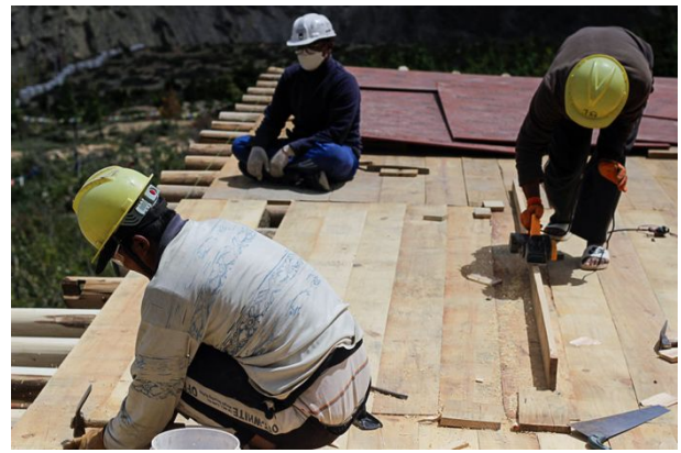
Figure 116: Placing the joist between the central beam and the balcony area.
