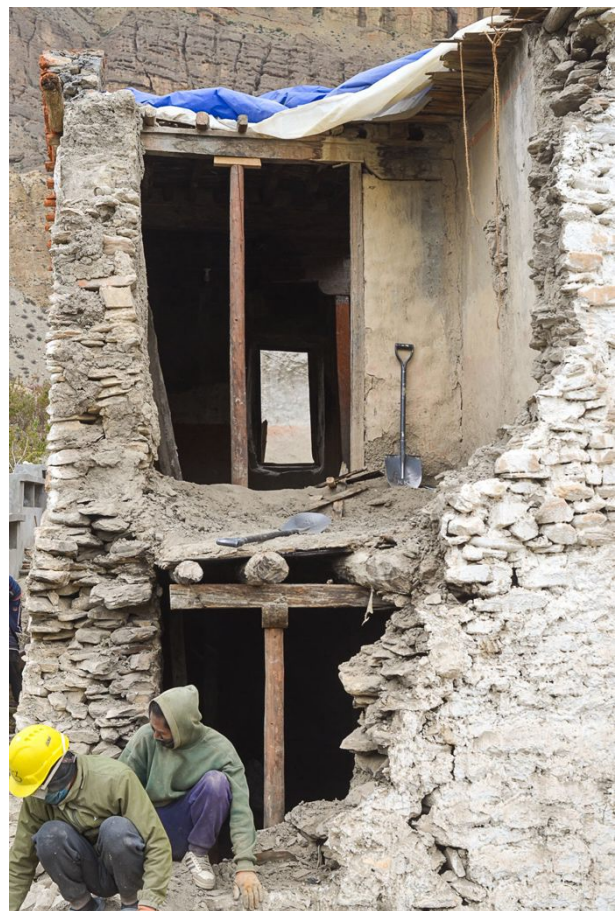
Figure 145: The walls at the corner turned out not to be structurally connected.
