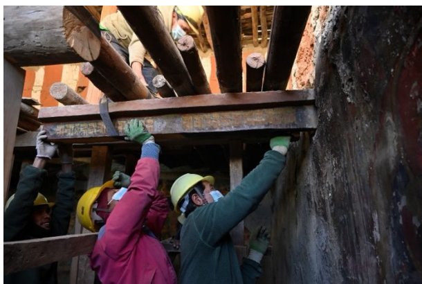
Figure 382: Removal of a painted beam of the upper level from the wall.
