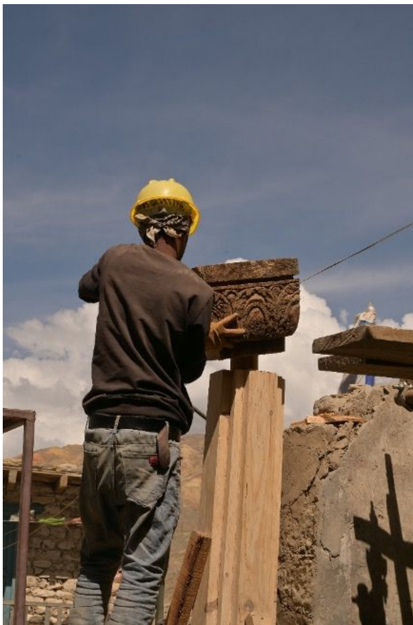
Figure 95: Connecting the old capital base to the new column.
