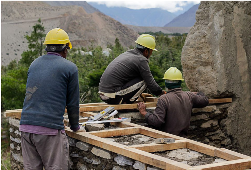
Figure 159: Laying a new wooden tie across the corner to connect the old and new stone walls.
