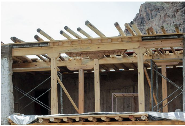
Figure 116: Placing the joist between the central beam and the balcony area.
