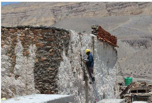
Figure 203: This worker undertakes repairs along the south wall of the monument. The southwestern corner in the foreground had to be repaired extensively.
