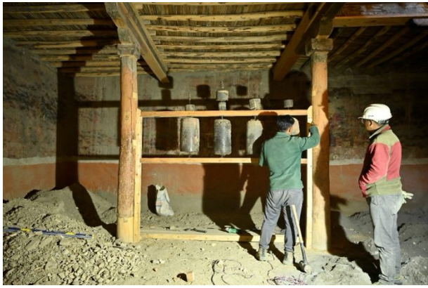
Figure 399: Reinstalling the old mani wheels in their original place.
