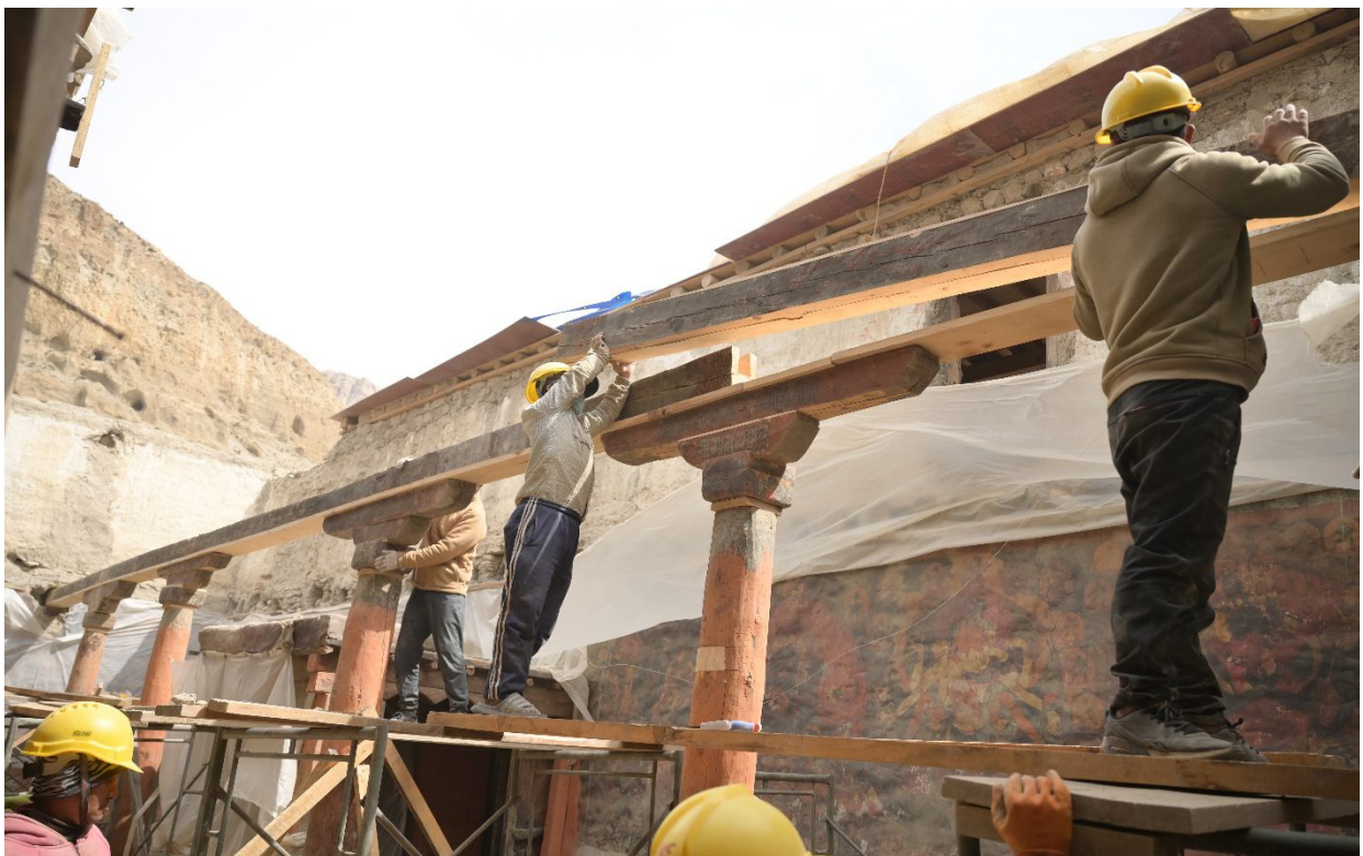
Figure 256: Reassembling the first row of pillars inside the Assembly Hall.
