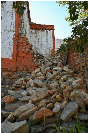
Figure 13: The structure to the right of the entrance partially collapsed in recent rains.
