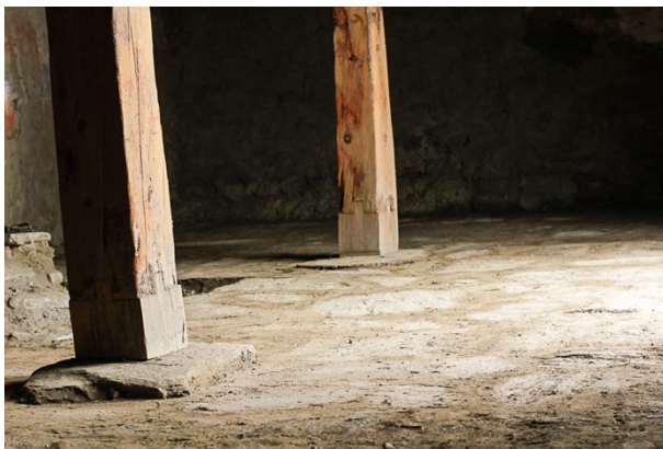
Figure 109: View of the Entry Hall's floor after completion, the base stone supporting the pillars slightly projecting from it.
