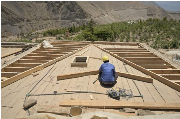
Figure 326: Constructing the wooden frame for the plywood with the sloping.
