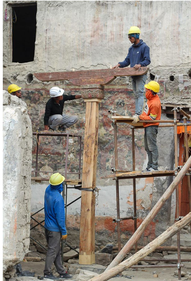
Figure 85: The original pillar, expanded in height, was joined with a new bedrock.
