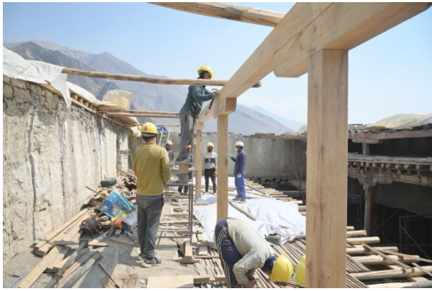
Figure 265: Reconstructing the upper floor above the first row of pillars.
