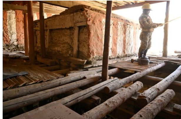
Figure 390: Removal of the mud on the third level around the lantern housing the uppermost part of the main image.
