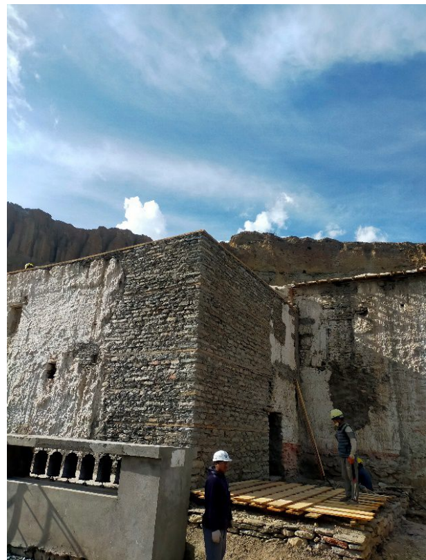
Figure 161: Once the corner wall was completed a stair was constructed to enable easy access the ground floor door.
