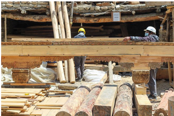
Figure 91: To fit the new and old parts together they were first assembled in the working area.
