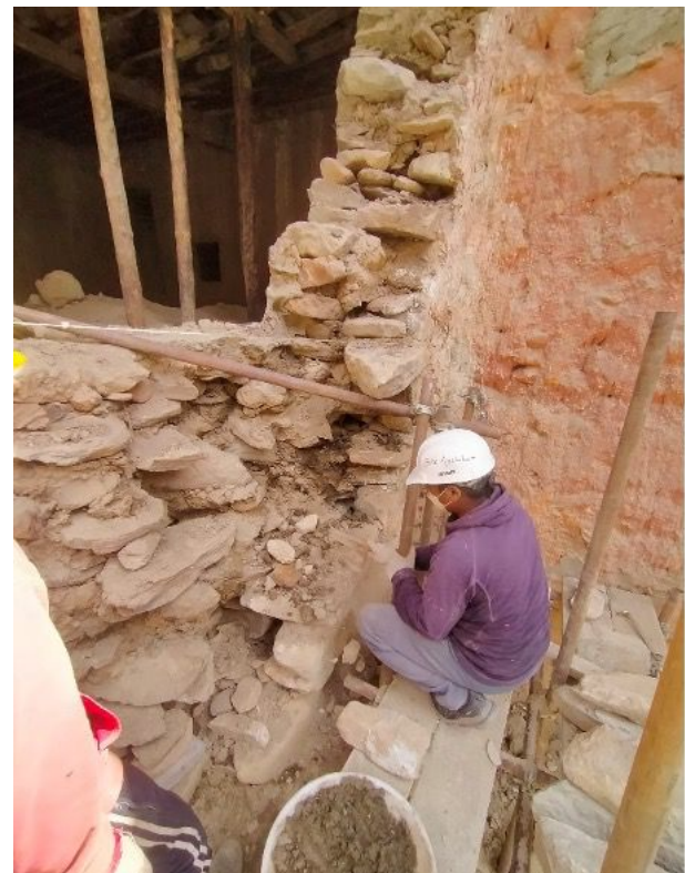
Figure 193: An extra wall was constructed in front of the problematic wall as support.
