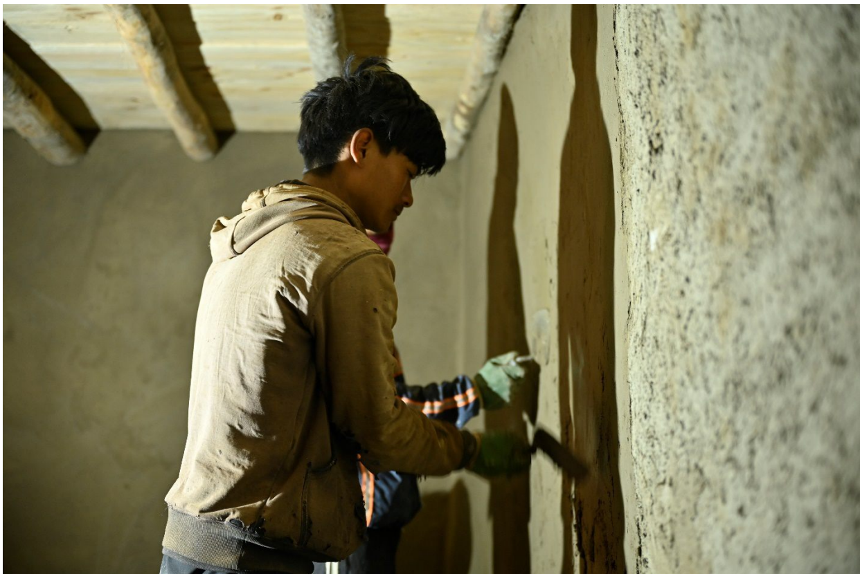
Figure 342: Applying fine plaster on the interior walls.
