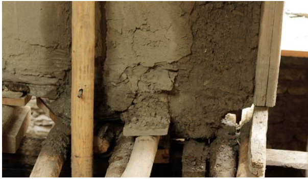
Figure 431: Rain damage to an exposed section of a wall which was later repaired again.
