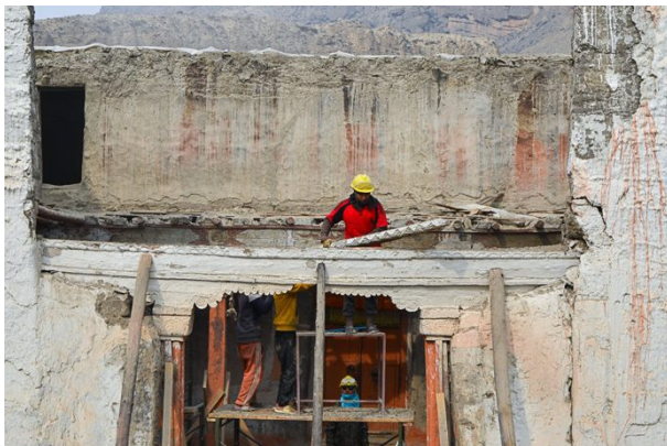
Figure 77: Then the porch was dismantled as well.
