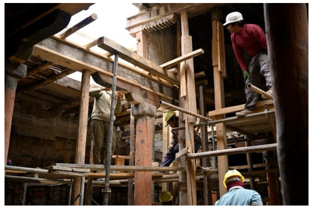
Figure 282: Reconstruction of the beam underneath the short wall on the other side of the same row three.
