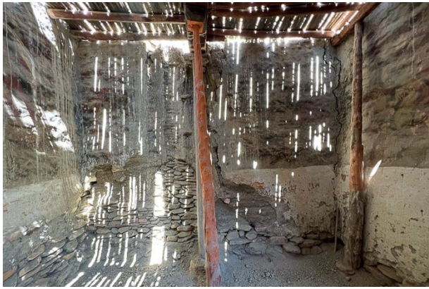
Figure 79: The severely damaged right-side wall of the Entry Hall during dismantling of the upper floor.
