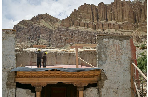
Figure 110: The area where the central beam is to be placed was strengthened by a leveled wooden plate.
