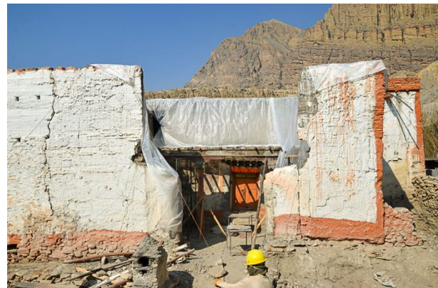
Figure 78: Once the entire interior structure of the Entry Hall was dismantled the wall paintings were protected with tarpaulin.
