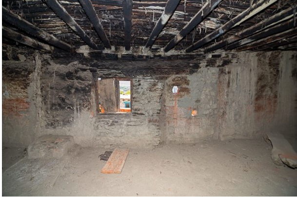
Figure 472: View of the balcony area before restoration, note the wooden members inside the wall.
