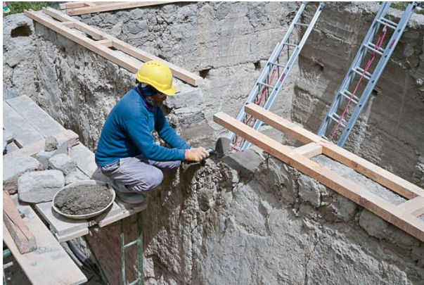
Figure 110: The area where the central beam is to be placed was strengthened by a leveled wooden plate.
