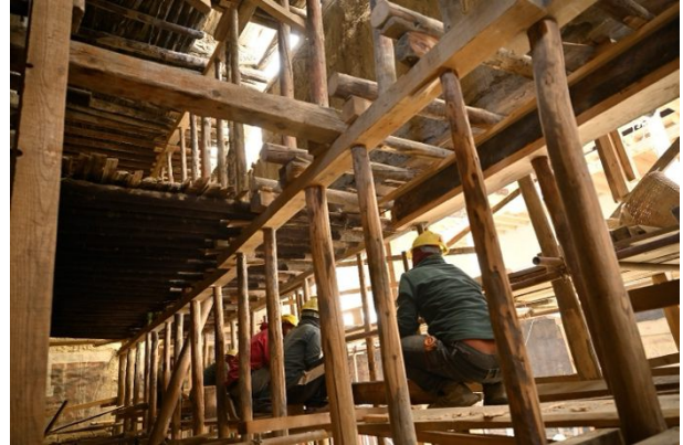
Figure 292: Preparing for the second beam to be placed underneath the painted wall.
