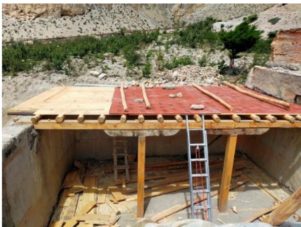
Figure 141: The structural wooden members for the roofing of the southwestern room prepared for assemblage.
