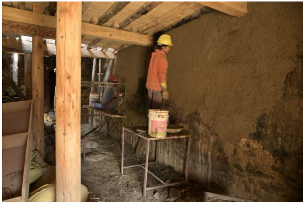
Figure 340: Plastering the interior of the ground floor of the South Wing.
