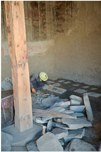
Figure 106: Laying the stone floor in the back corner of the Entry Hall.
