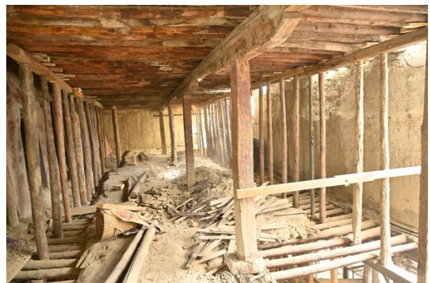
Figure 284: Preparation of the restoration of rows four and five by installing additional supports.
