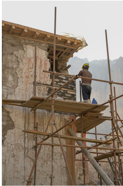
Figure 125: Placing the lowest wall tie on the upper floor of the northeast corner.
