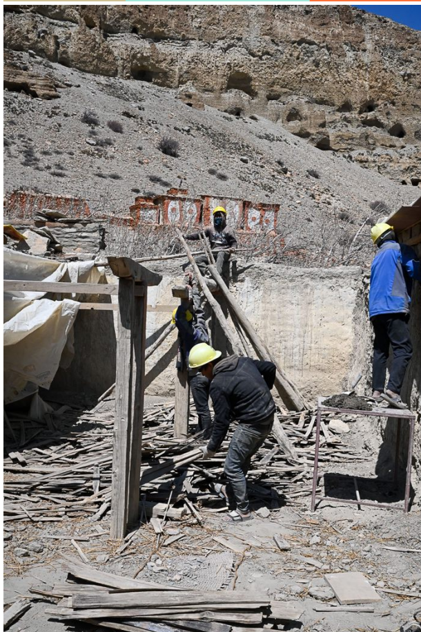
Figure 245: Dismantling the support structure on the upper level.
