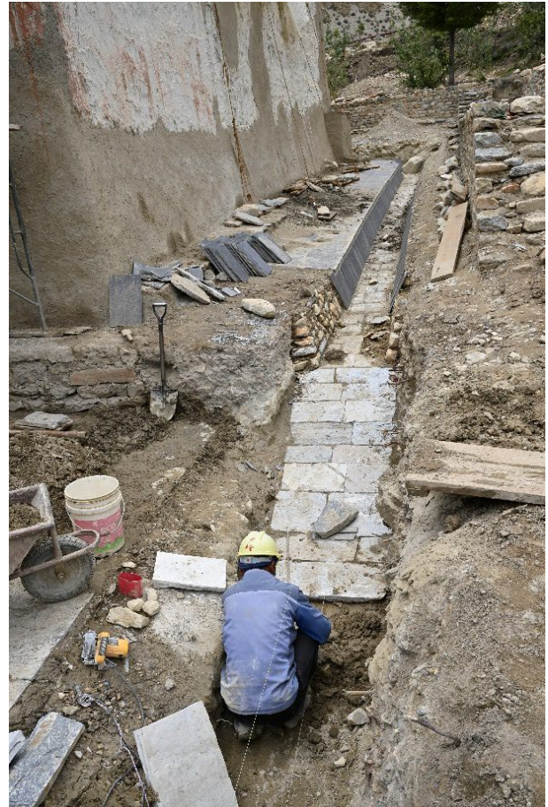
Figure 56: Paving the drainage with stone slates, first along the ground, then along the reinforced slopes.
