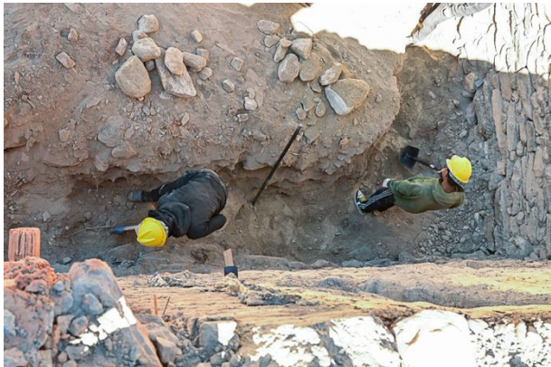
Figure 59: All along the outer wall of the monument a ditch was dug for the wall strengthening the foundation.
