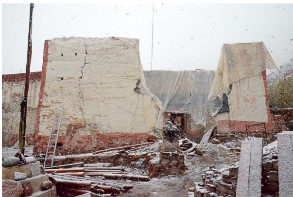
Figure 430: In late April 2023 snowfall interrupted the work. At that time the Entry Hall with its murals were protected by the tarpaulin sheets to prevent damage.
