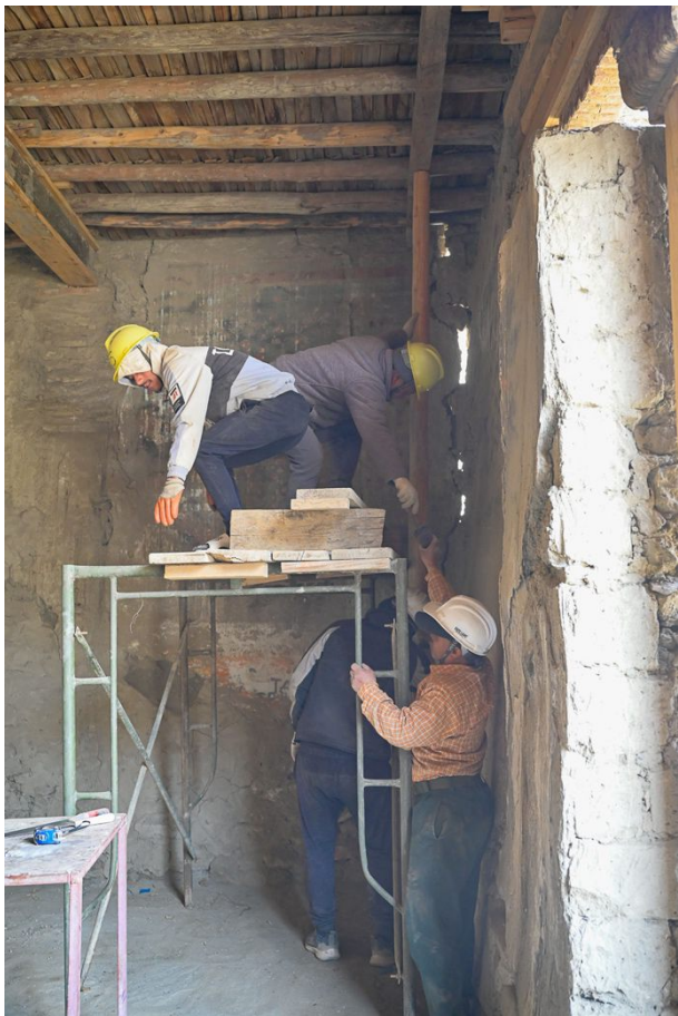
Figure 122: Supporting the cross beams of the northeast corner on the ground floor level.
