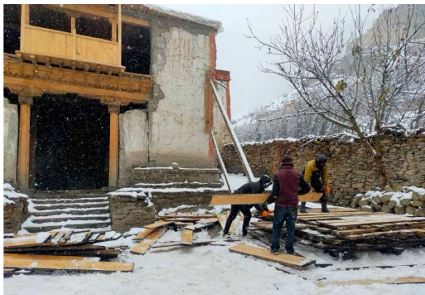
Figure 221: Stacking the wood properly.
