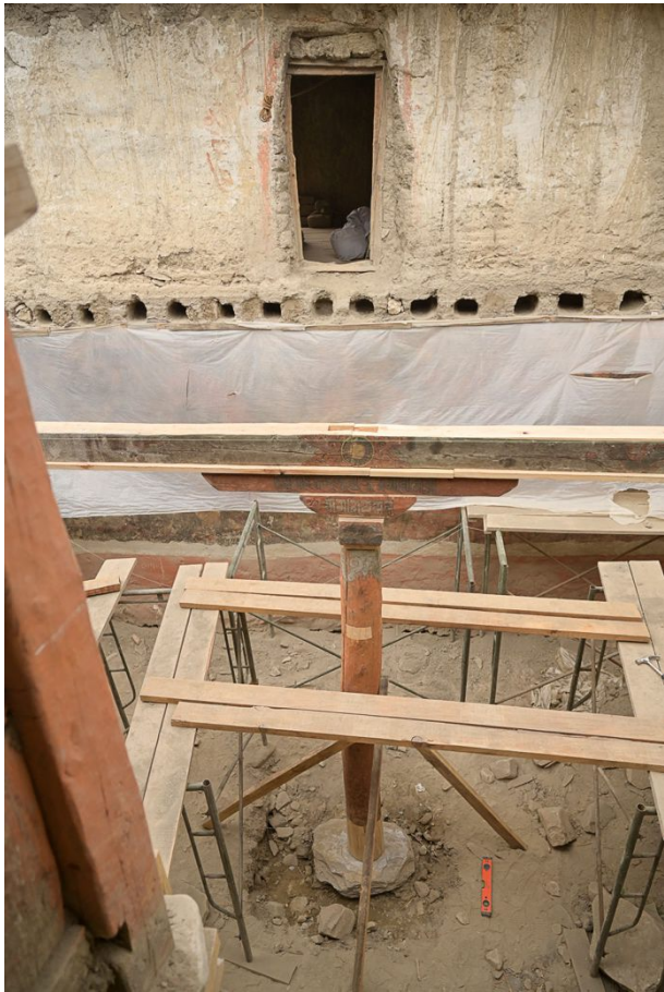
Figure 257: View of one pillar reassembled with its capital and beam, all parts joined to each other for seismic strengthening.
