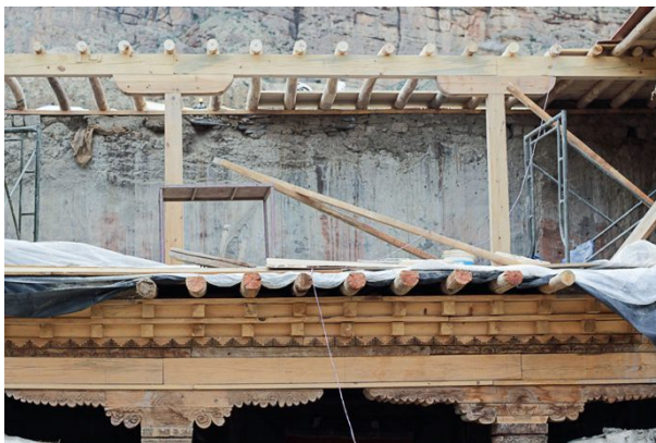
Figure 114: Detail of the partial reconstruction with the back joists in place.
