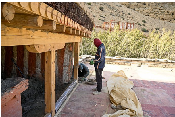
Figure 363: Completing the plywood sheeting and sealing off the area above the sanctum.
