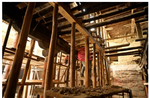
Figure 271: Inserting new joists into holes at a higher level of the painted wall.
