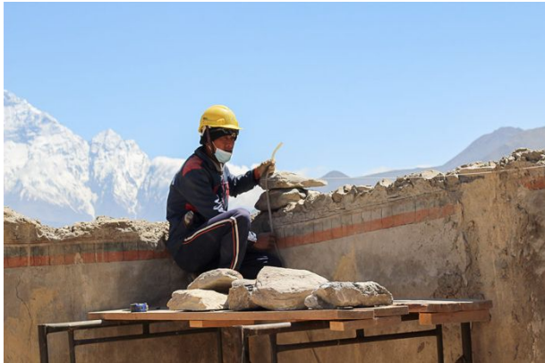
Figure 137: Leveling the top of the wall to enable the installation of wall ties for seismic strengthening.
