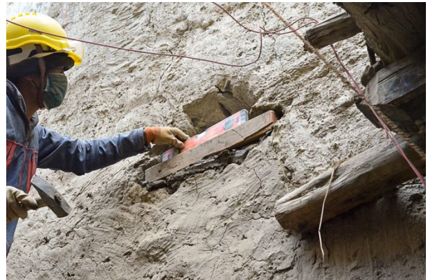
Figure 81: The original post holding the porch was lengthened by adding a new bottom section.
