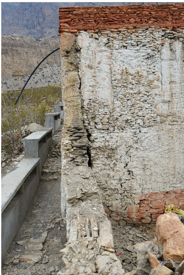
Figure 145: The walls at the corner turned out not to be structurally connected.
