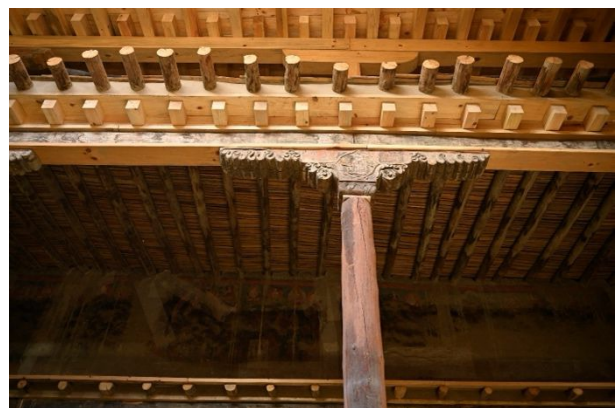
Figure 307: Reassembling the superstructure above the intermediate roof covering the painted wall area.
