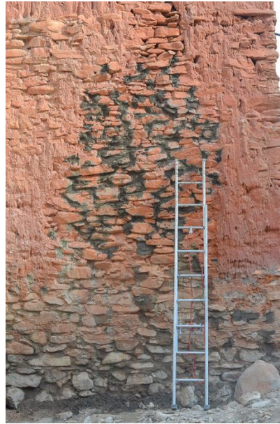
Figure 204: Here an area of loose stones was relayed.
