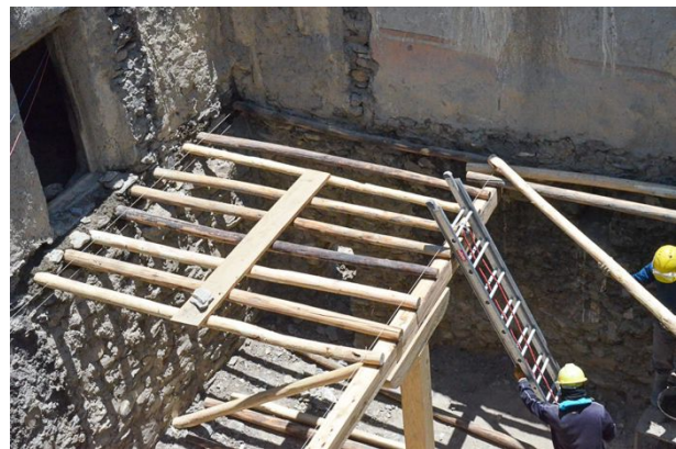
Figure 135: The new beam was placed on a new wooden support inside the wall.
