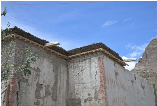
Figure 353: Parapet with Perma and waterspouts installed on the entrance side of the temple.
