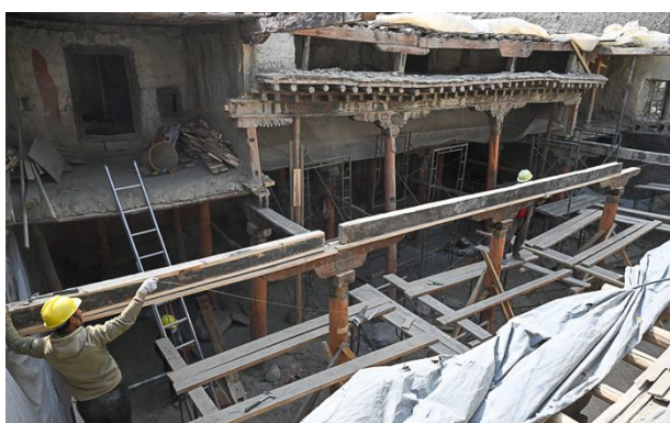
Figure 263: Rebuilding row two on ground level on April 18.
