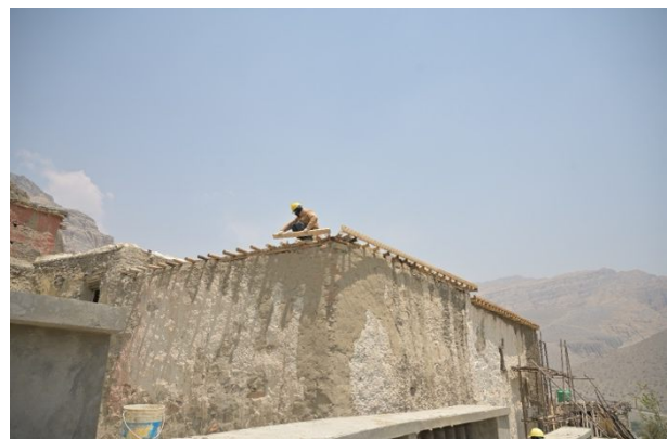
Figure 325: Placing the decorated wooden frieze at the bottom of the parapet.
