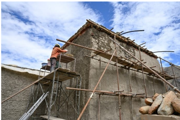
Figure 209: Wall repairs and plastering on the exterior of the temple.
