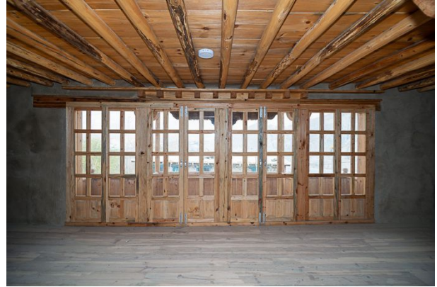
Figure 472: View of the balcony area before restoration, note the wooden members inside the wall.
