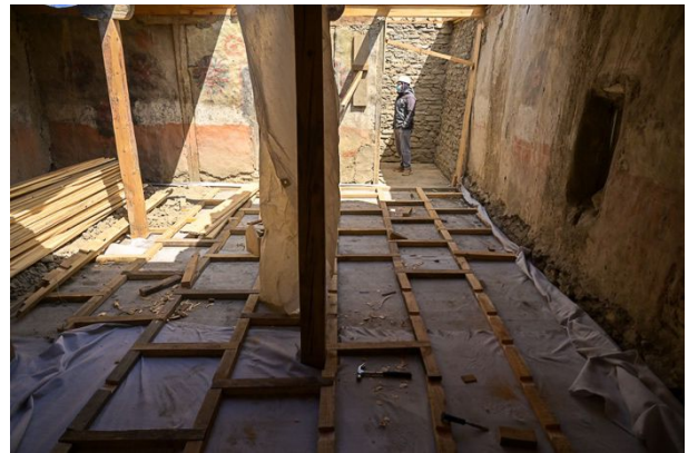
Figure 182: Preparing the wooden floor for the painted room of the south wing.
