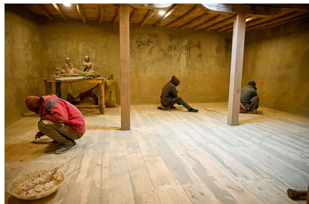
Figure 408: Fine plaster was applied to all the undecorated walls of the upper floor.
