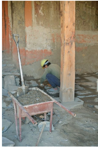
Figure 106: Laying the stone floor in the back corner of the Entry Hall.
