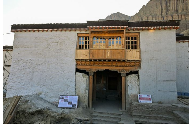
Figure 422: The patched-up crack in the entry wall before the installation of wall ties. Note that the balcony door is still without glass.
