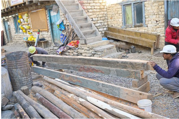
Figure 248: Inspecting the original wooden beams to prepare them for reuse.
