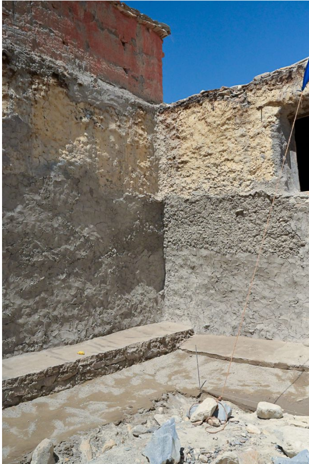
Figure 64: Covering the foundation support wall and the ground in front of it with mud.
