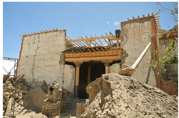
Figure 112: The wooden structure and the joists of this room are entirely replaced, as the best original wooden members were used for the lower floors to retain their original appearance.
