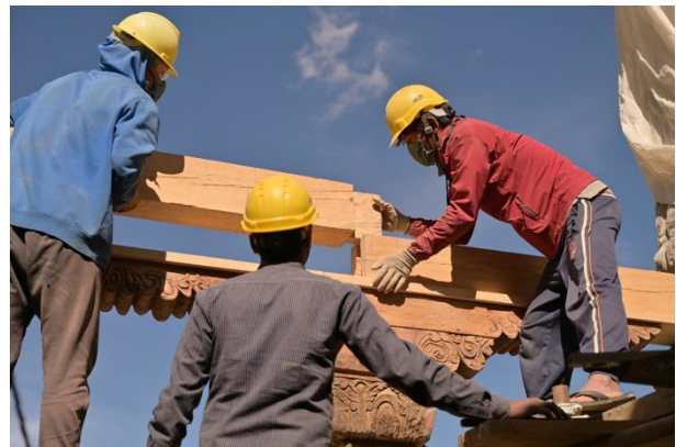
Figure 98: Arranging the positioning of the central beam as per measurements.
