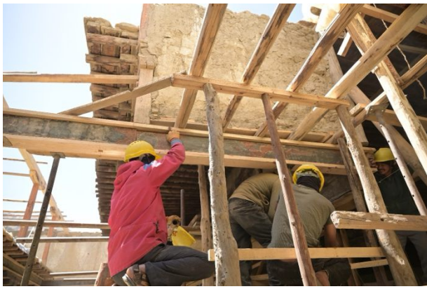
Figure 280: Another perspective of the process of reinserting the restored beam underneath the short side of the painted wall.
