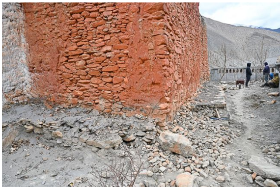
Figure 43: Clearing along the foundation of the temple.
