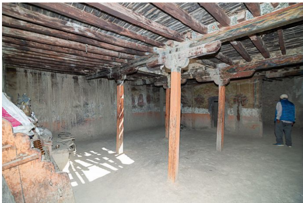
Figure 474: View of the painted room before restoration.
