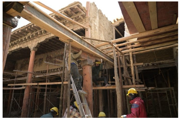
Figure 280: Another perspective of the process of reinserting the restored beam underneath the short side of the painted wall.
