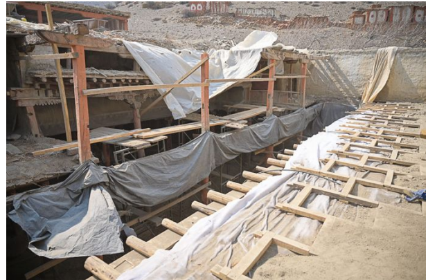
Figure 259: Creation of floor frame for the first bay while the roof above the third bay is being dismantled on April 11.
