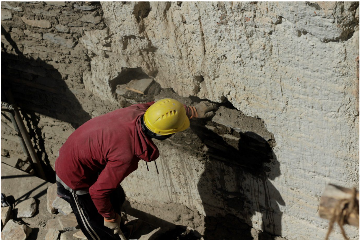
Figure 208: View from top during the repair of a stone wall showing wooden members to connect the repair to the original wall.
