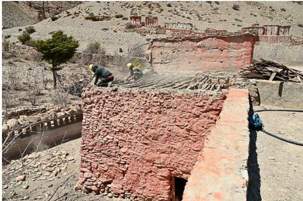
Figure 37: The structure to the south side of the apse clearly is a later addition and poorly constructed.
