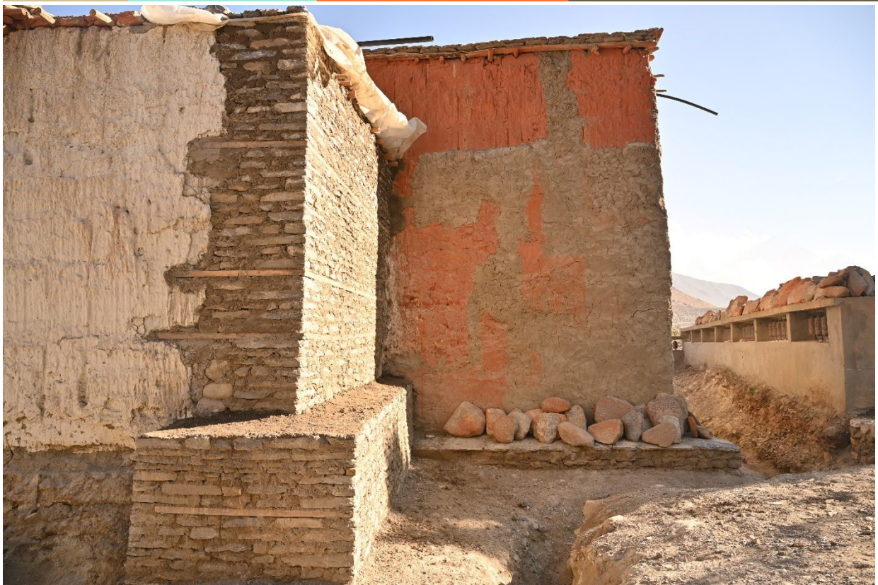
Figure 202: Northwest corner wall after completion.
