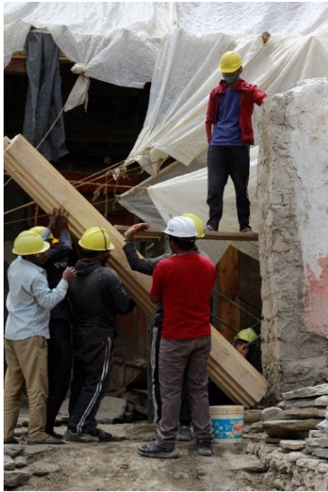
Figure 93: Placing the front column on the bed stone with a projection connecting it to it.
