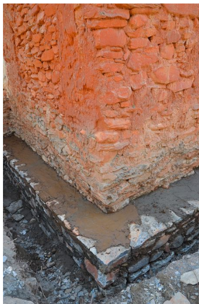
Figure 61: The a stonewall was constructed along the building to consolidate its foundation.
