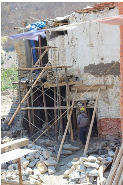
Figure 150: The east side of the corner with temporary supports added while preparing the foundation of the new wall.
