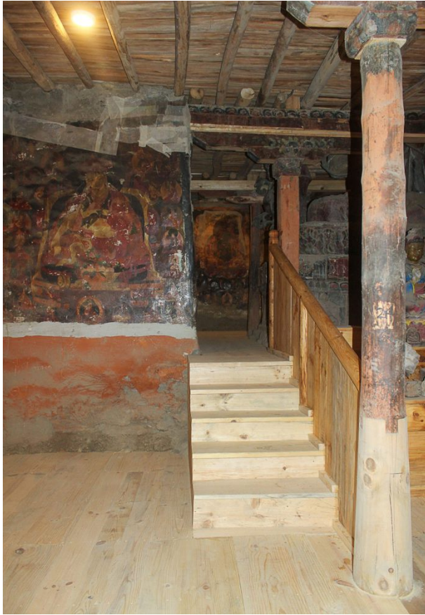
Figure 419: Stairs to the Ambulatory around the main image of Buddha Maitreya after restoration.
