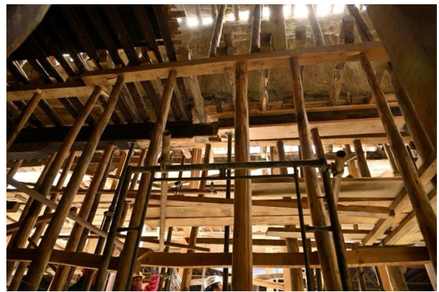
Figure 293: Workers ready to lift the second beam into its place underneath the painted wall.
