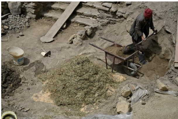
Figure 25: Preparing the mud mixture with hay and straw for the mud-bricks and rough plaster.
