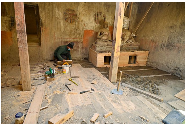
Figure 406: Finishing the flooring in the painted room around the two statues located there in early October.
