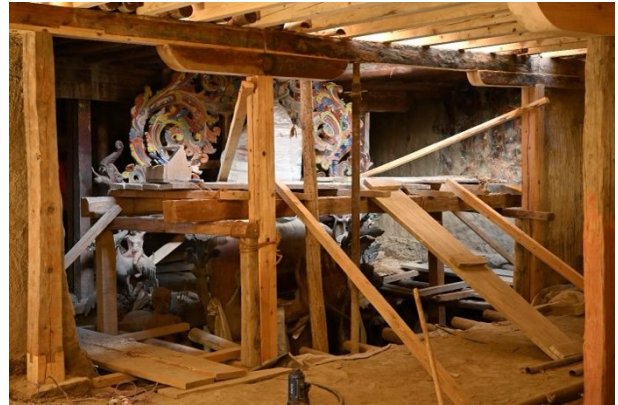
Figure 374: The upper-level area in front of the main sculpture after the main beam has been restored.
