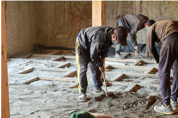
Figure 119: Laying out the wooden batten to hold the flooring; with the hollow space filled with mud.
