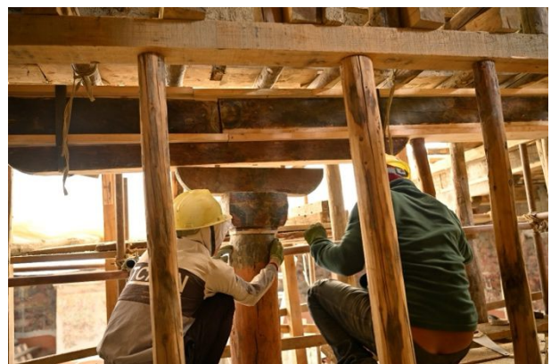
Figure 296: Placing the pillar in its original place, now supported by a solid foundation and connected across all parts.
