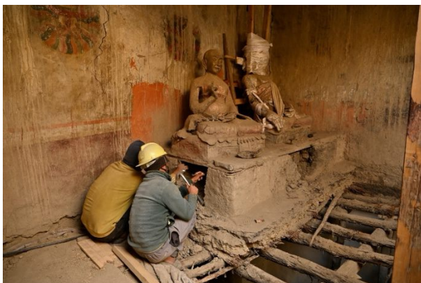
Figure 183: Cutting into the mud pedestal of the sculptures to be able to support them from below.
