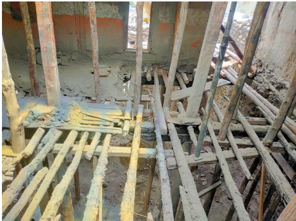
Figure 167: View of the painted room after removing its floor to enable the replacement of the wooden structure underneath.
