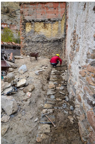
Figure 61: The a stonewall was constructed along the building to consolidate its foundation.
