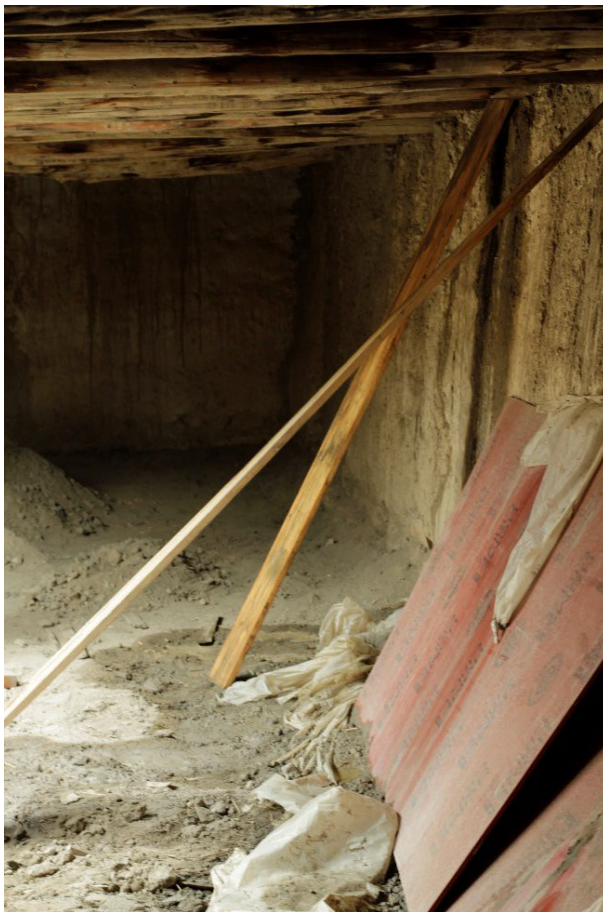
Figure 433: Plastic sheets and plywood used to prevent water affecting the wall paintings on the floor underneath.
