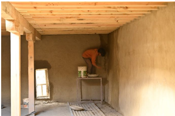
Figure 402: Application of the final mud plaster on the walls of the upper level.
