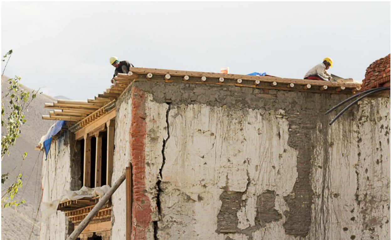
Figure 118: Placing the wooden members with circle design along the top of the wall to support the parapet.
