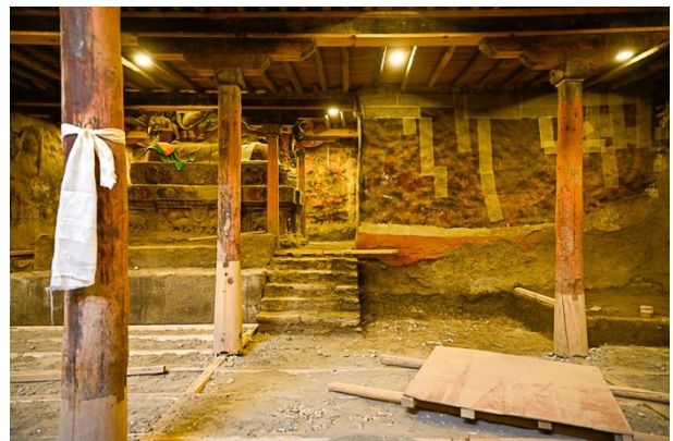
Figure 415: Installing the wooden frames for flooring the Ambulatory around the Maitreya sculpture. Note the massive flight of stairs installed at that stage.
