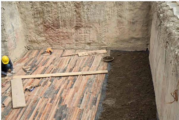
Figure 102: Between the wood splits and the mud layer a breathing fabric was added to reduce dust.
