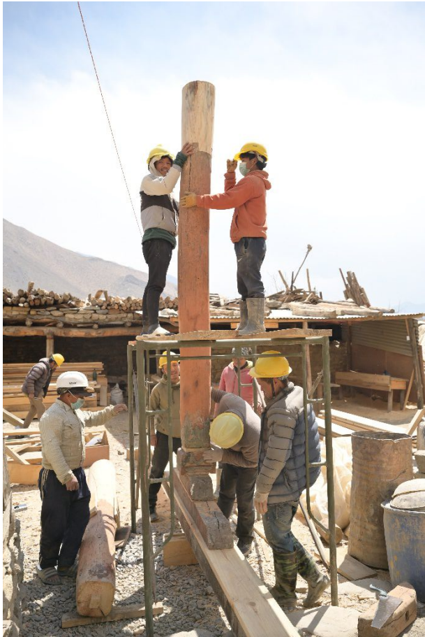
Figure 254: To ensure structural stability joints were created between each part of the capitals.
