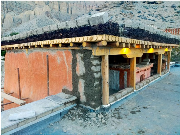
Figure 395: Repairing the side of the third-floor extension above the sanctum.
