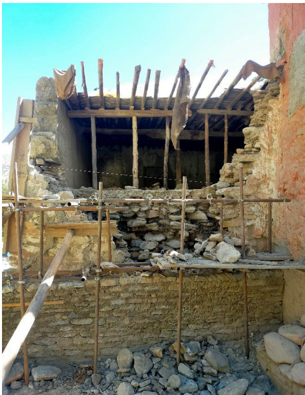
Figure 193: An extra wall was constructed in front of the problematic wall as support.
