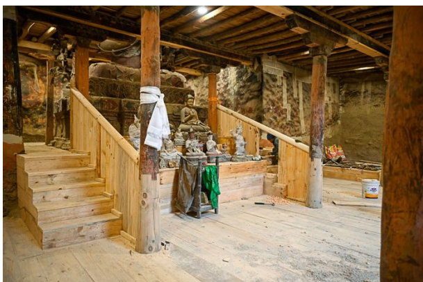
Figure 416: The same area of the Assembly Hall with the stairs reduced and wooden frames for the floor in the Assembly Hall installed.
