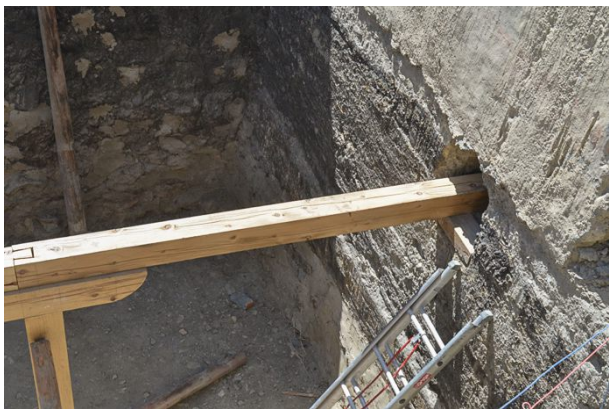
Figure 135: The new beam was placed on a new wooden support inside the wall.
