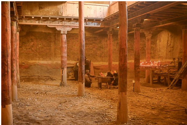
Figure 413: Villagers working on leveling the floor of the Assembly Hall.
