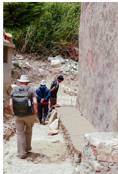
Figure 61: The a stonewall was constructed along the building to consolidate its foundation.
