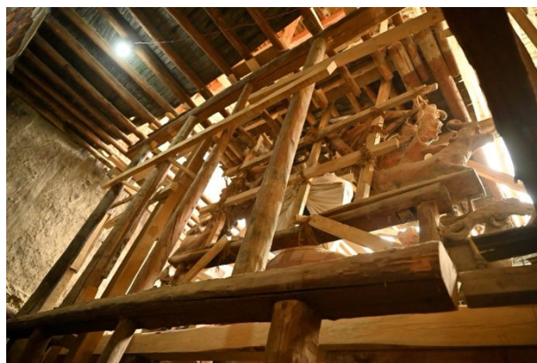
Figure 381: Detail showing the attachment of the support through pegs and ropes.
