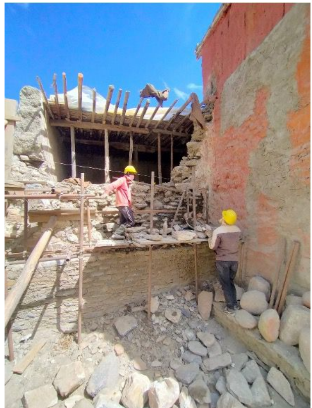
Figure 196: Construction of the new wall along the lower section of the wall and connecting it with the old one.
