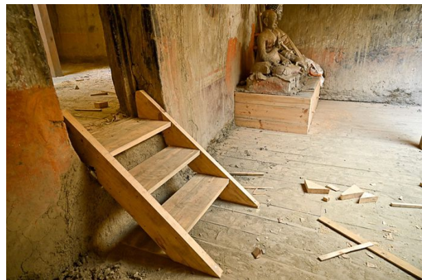
Figure 406: Finishing the flooring in the painted room around the two statues located there in early October.
