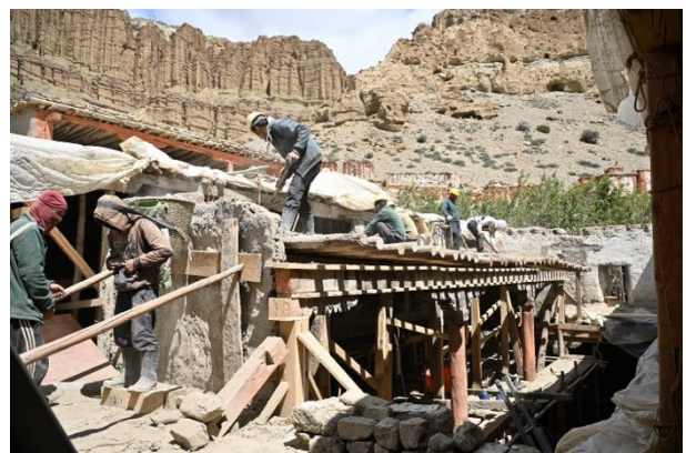
Figure 301: Continuing to reassemble the original structure supported by the long pillars.
