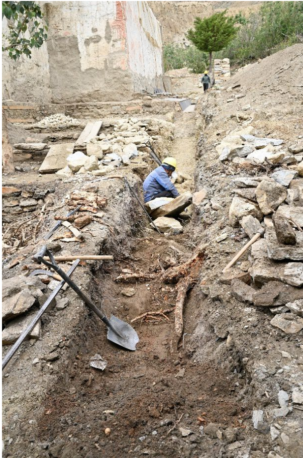
Figure 55: Digging the drainage on the northeast of the monument.
