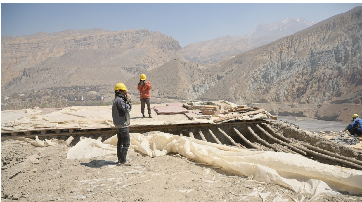
Figure 244: Removal of the roof above the Assembly Hall, including the plastic sheets added in an earlier village restoration.
