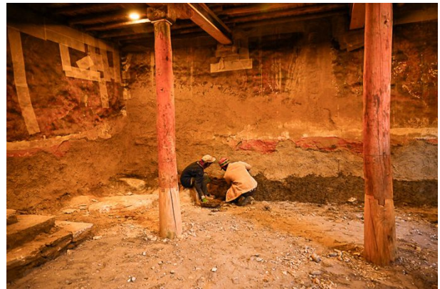
Figure 414: Workers applying rough plaster along the bottom of the wall in the southwest corner of the Assembly Hall. Note the stone bolder projecting in this area.
