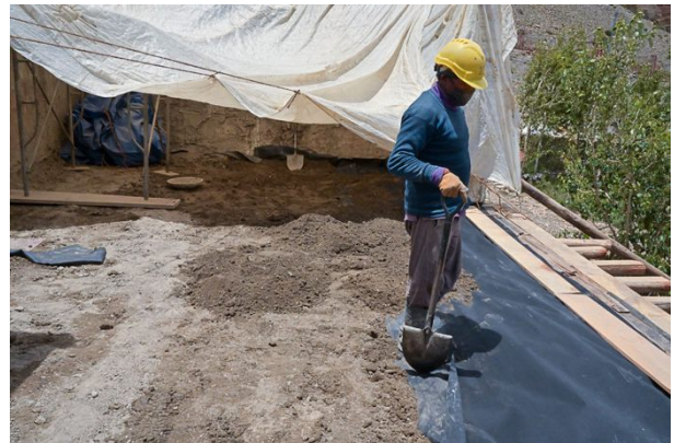
Figure 102: Between the wood splits and the mud layer a breathing fabric was added to reduce dust.
