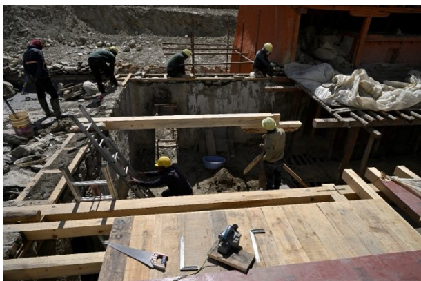
Figure 358: Installing wooden ties along the top of the Assembly Hall wall.
