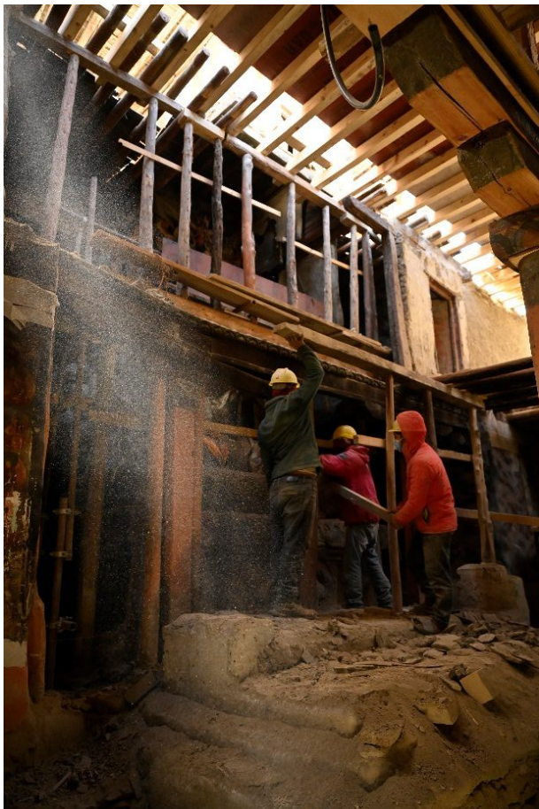
Figure 369: Mounting the supports in front of the main image.
