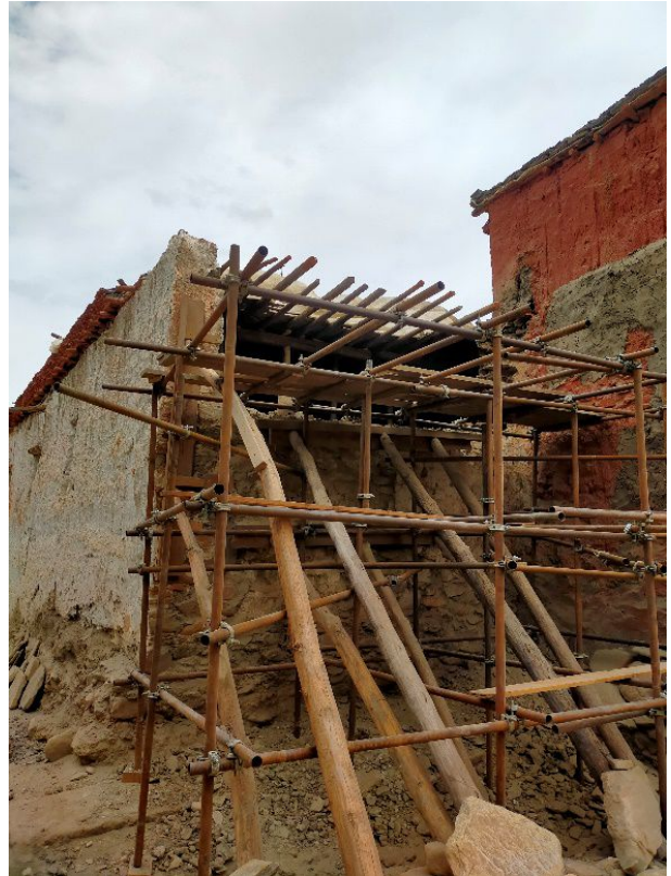
Figure 191: First the wall was shored up to prepare the dismantling from the top.
