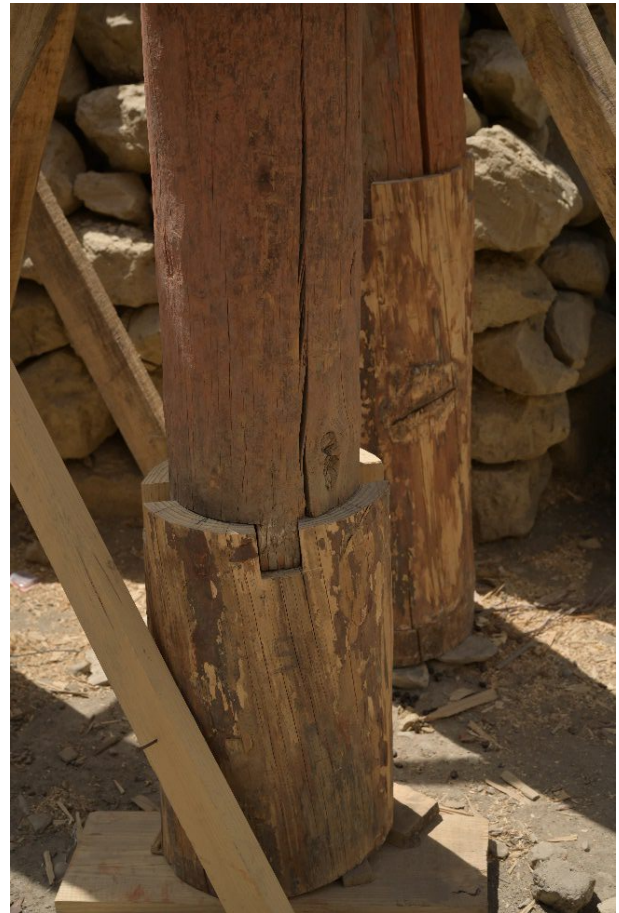
Figure 250: Once the structure was taken down the rotten bottom parts of the pillars were replaced.
