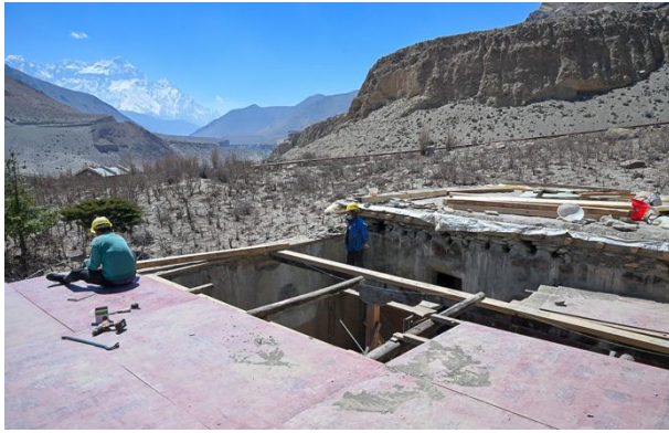
Figure 179: Removing the temporary roof of the south wing.
