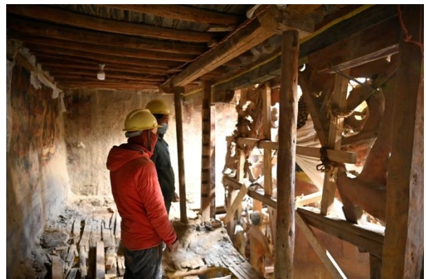
Figure 379: Placing additional supports to the back of the main sculpture to enable the restoration of the broken beam.
