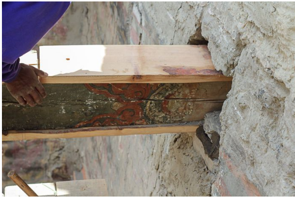
Figure 89: On the wall sides the reassembled beam was placed on a leveled stone plate inside the wall.
