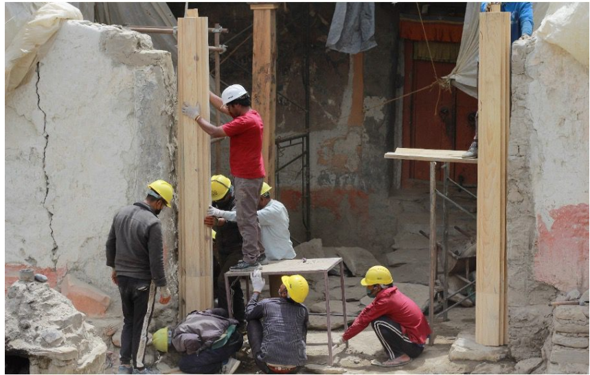
Figure 93: Placing the front column on the bed stone with a projection connecting it to it.
