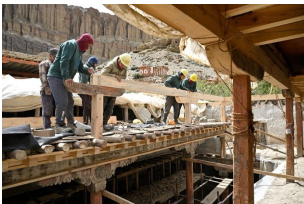
Figure 307: Reassembling the superstructure above the intermediate roof covering the painted wall area.
