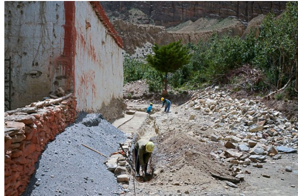
Figure 45: A worker digging the drainage channel at a distance to the temple's walls.
