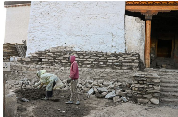
Figure 424: The stairs constructed between the entrance to the compound and the monastery courtyard.
