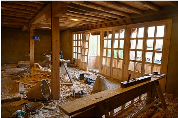
Figure 130: The balcony door has many compartments for glass panels and thus was a complex work.
