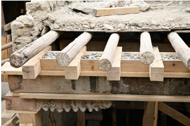
Figure 303: Rebuilding the structure above the reassembled beam following the original construction.
