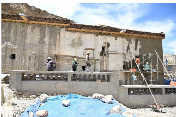
Figure 344: Repairing and plastering the outside wall of the South Wing.
