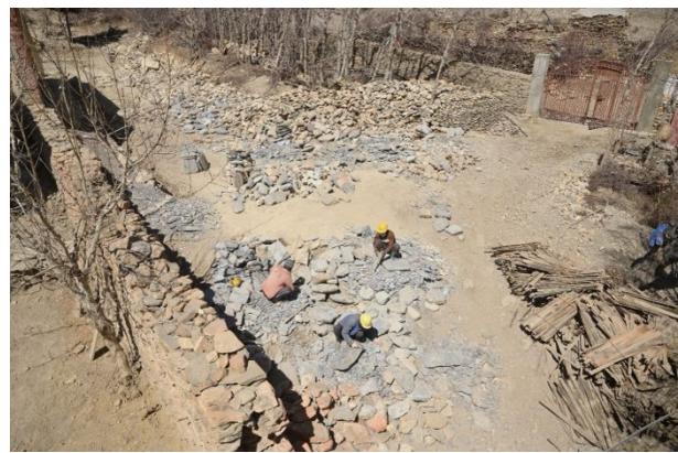
Figure 47: Foundation support and drainage at the back of the temple in October 2023.
