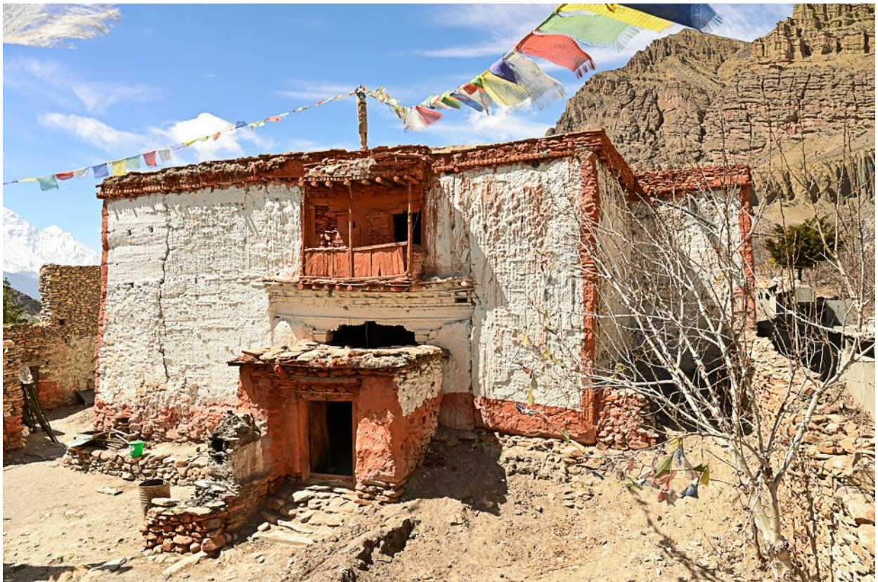
Figure 74: The temple on March 29, 2023, after clearing but before work started on the Entry Hall of the building.
