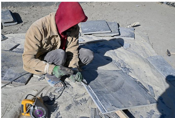
Figure 367: Cutting an overlap into the edge of the stone slate.
