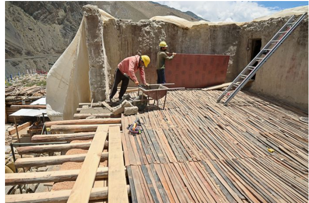
Figure 101: The old wood splits were screwed to the joists and retain the previous appearance of the Entry Hall ceiling.
