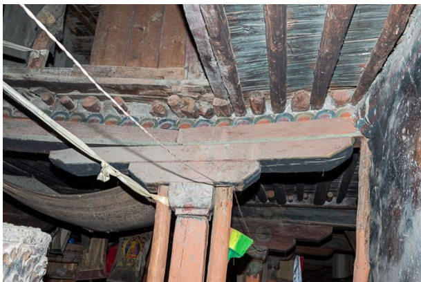
Figure 458: View of the distortion of the wooden structure due to the sagging of a pillar immediately in front of the main Buddha image.
