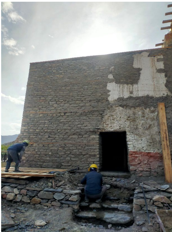
Figure 161: Once the corner wall was completed a stair was constructed to enable easy access the ground floor door.
