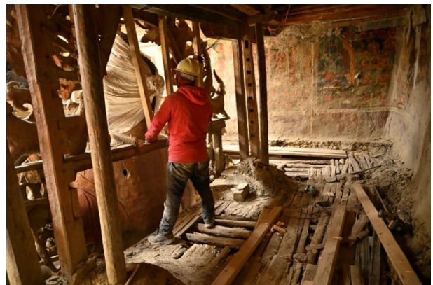
Figure 376: Removal of the frame behind the main image's head to expose the broken beam in this area.
