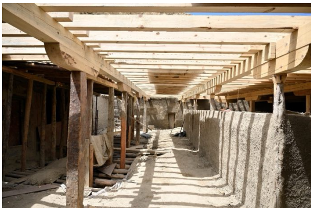
Figure 316: The area between the painted wall (right) and the main sculpture after finishing the wooden structure.
