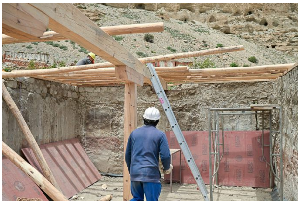
Figure 112: The wooden structure and the joists of this room are entirely replaced, as the best original wooden members were used for the lower floors to retain their original appearance.
