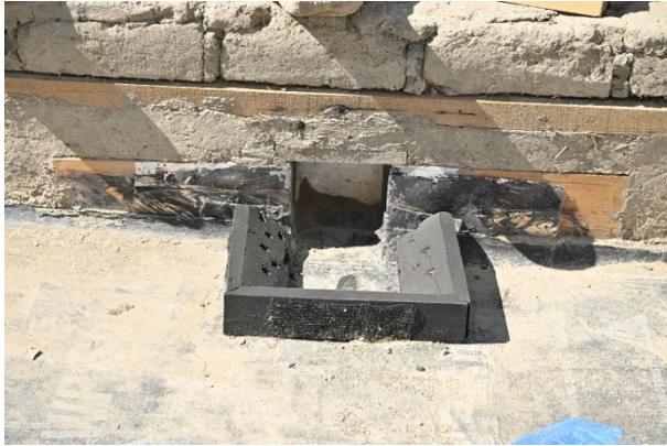
Figure 332: Wooden barrier around the waterspout.
