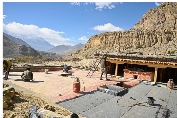
Figure 363: Completing the plywood sheeting and sealing off the area above the sanctum.
