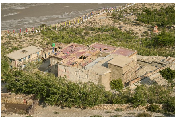
Figure 357: View of the site during the restoration in June 16.
