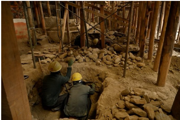
Figure 309: Excavating the pillar foundations after dismantling while the fourth-row pillars are still in place.
