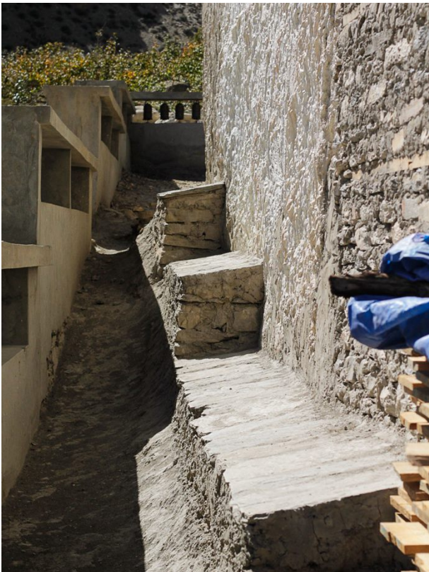
Figure 69: Along the south side the foundation wall had to be stepped.
