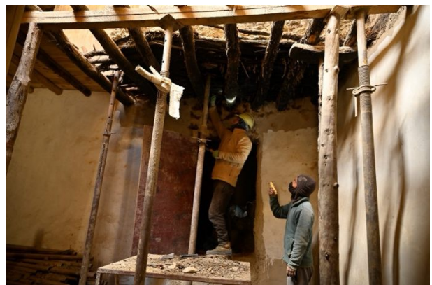
Figure 183: Cutting into the mud pedestal of the sculptures to be able to support them from below.
