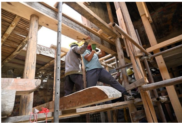
Figure 282: Reconstruction of the beam underneath the short wall on the other side of the same row three.
