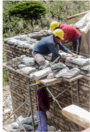
Figure 159: Laying a new wooden tie across the corner to connect the old and new stone walls.
