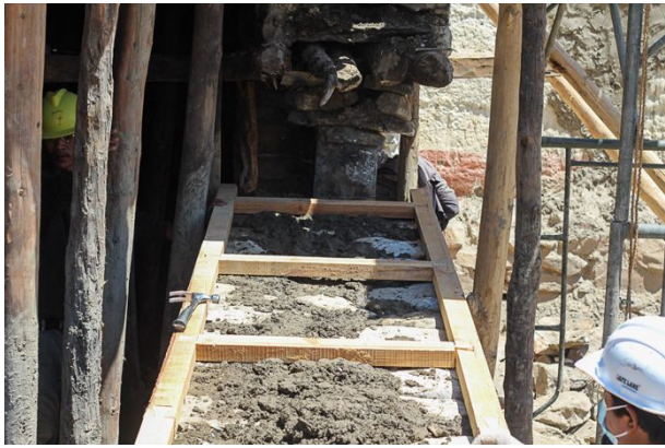
Figure 153: Wooden wall ties were added to the wall for seismic strengthening.
