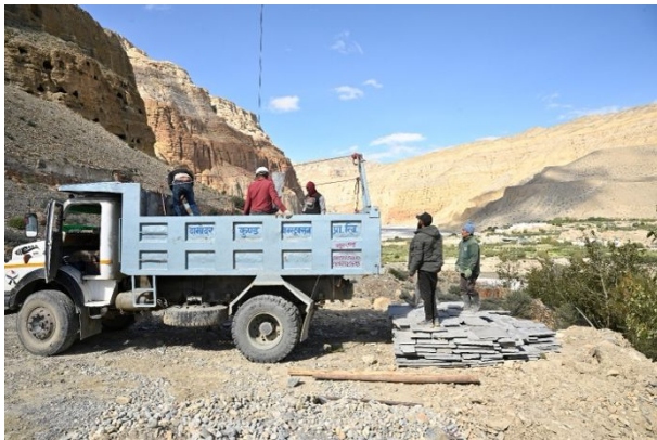
Figure 28: Construction truck delivering the stone slates.
