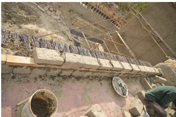
Figure 330: Construction of the traditional parapet with the apple twig bundles on the outside.
