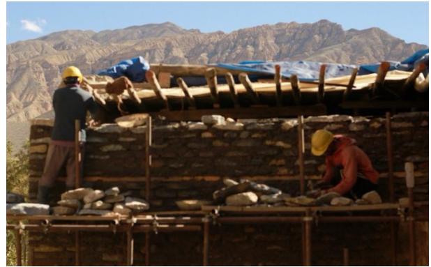
Figure 198: The wall reconstructed to the level of the first floor, where a wall-tie was inserted.
