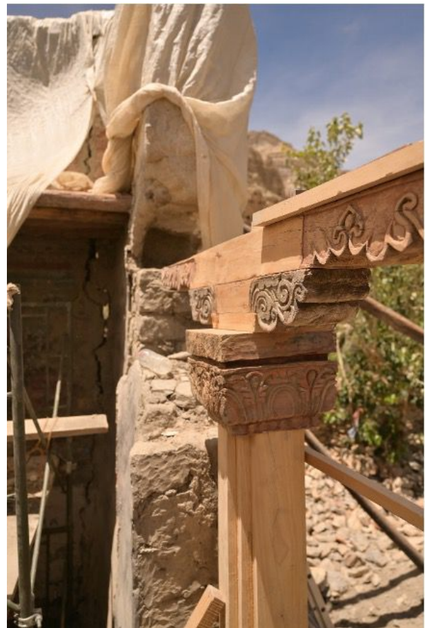
Figure 94: Checking the placement of the new columns with small wooden connectors.
