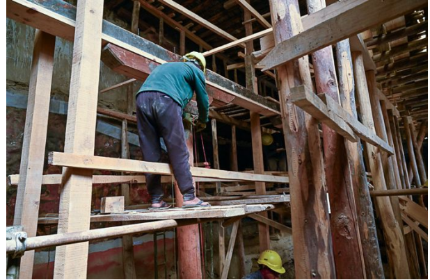
Figure 313: Reinstalling the repaired and strengthened beam in its original place.
