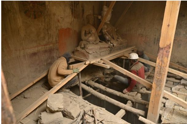
Figure 185: Installing supports from the sides to keep the sculptures in place.
