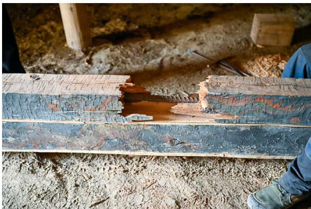
Figure 310: Reassembling the broken beam with an iron rod.
