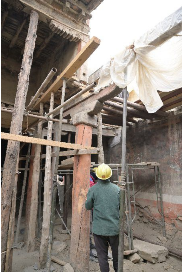
Figure 274: Preparing to take out the pillar underneath the corner of the painted wall in the third row.
