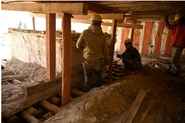
Figure 390: Removal of the mud on the third level around the lantern housing the uppermost part of the main image.
