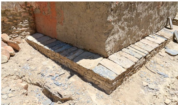
Figure 66: The foundation support wall after laying the stone slate upon the mud layer.
