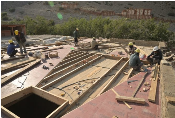
Figure 351: Roof work above the Entry Hall.
