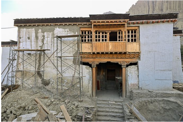
Figure 422: The patched-up crack in the entry wall before the installation of wall ties. Note that the balcony door is still without glass.
