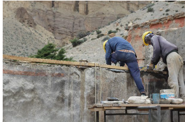
Figure 137: Leveling the top of the wall to enable the installation of wall ties for seismic strengthening.
