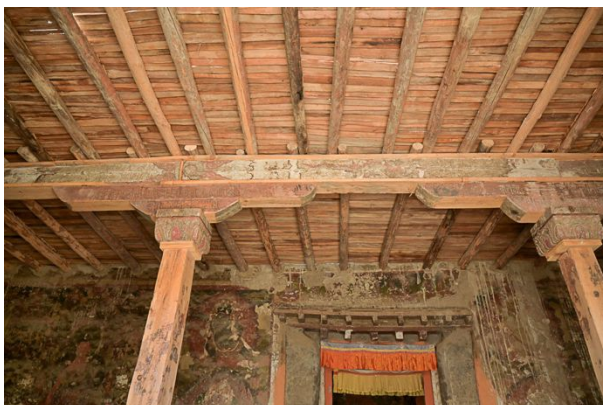
Figure 104: View of the ceiling of the Entry Hall after placing original wood splits on the joists.
