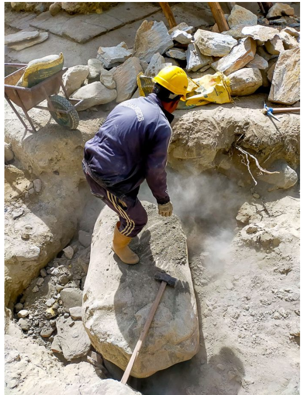
Figure 70: Work on the foundation and drainage was difficult as big boulders were occasionally in the way.
