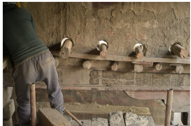
Figure 271: Inserting new joists into holes at a higher level of the painted wall.
